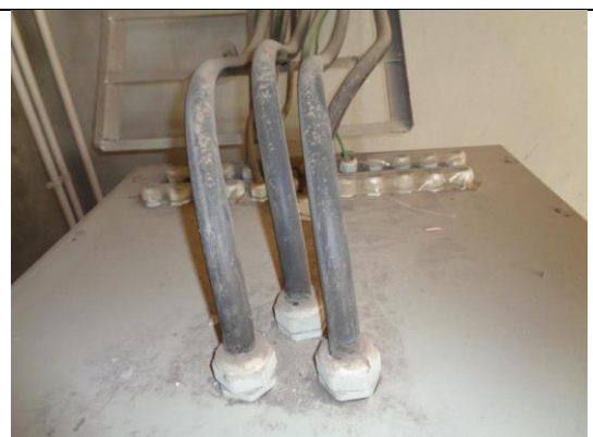
Cable entry is done through cable gland with base/top plates.
