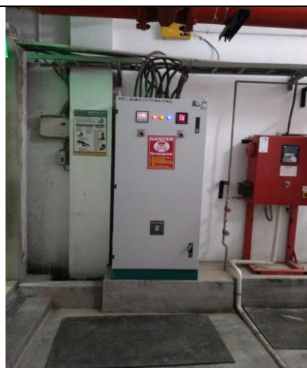
Typical cable entry system into electrical panel in floors
