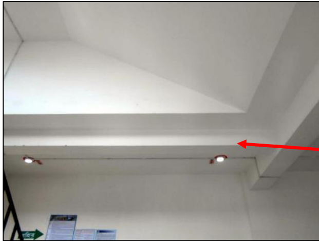
Extra beam on stair
