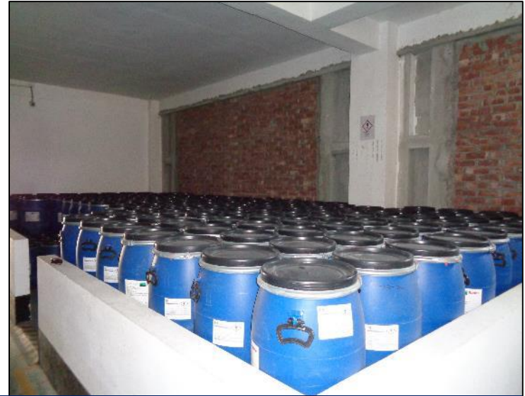
Excessive Loading on the ground floor and 1 st floor
