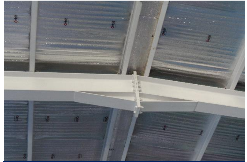
Rafter to rafter connection
