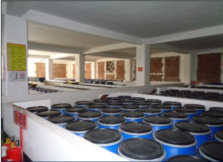
Excessive Loading on the ground floor and 1 st floor
