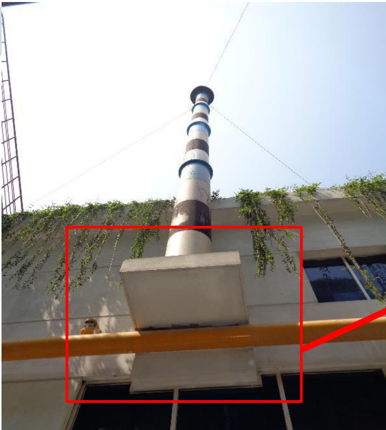
Chimney resting on corbel (east side)
