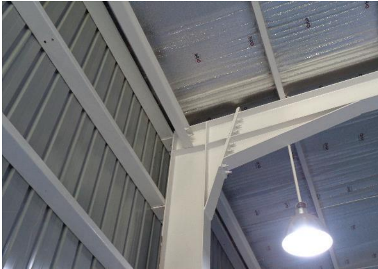
Rafter to column connection
