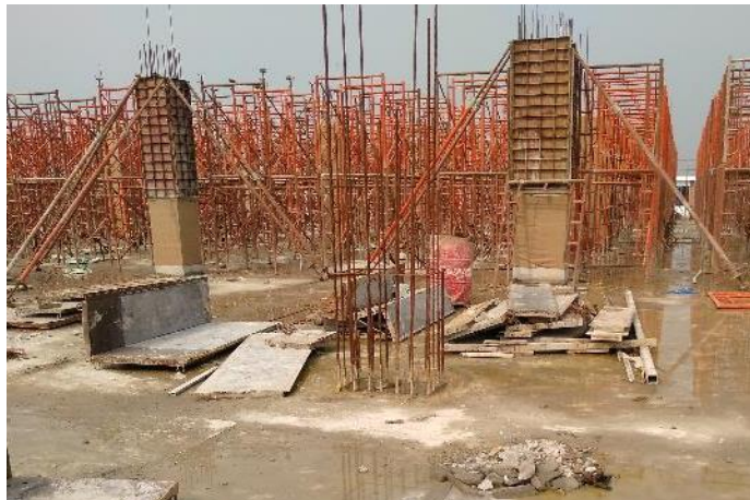
Rebar in L-shaped column
