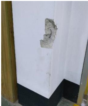
Additional column confirmed by scanning
