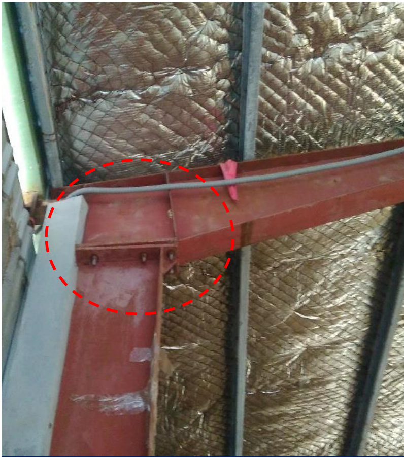
Gap between connections plates
