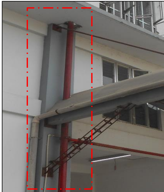
Porch connected to the wall of the buildings
