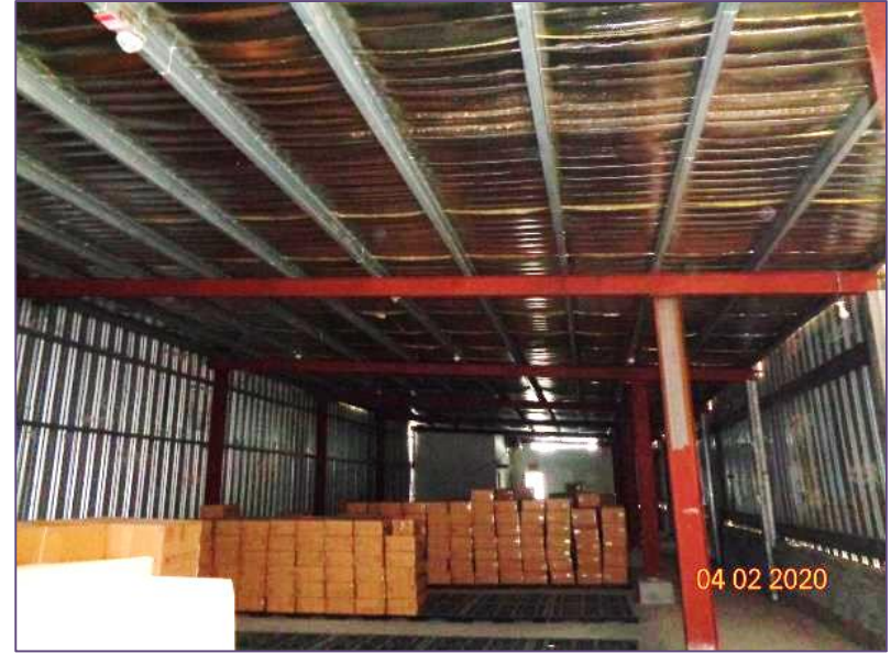
Interior of steel shed
