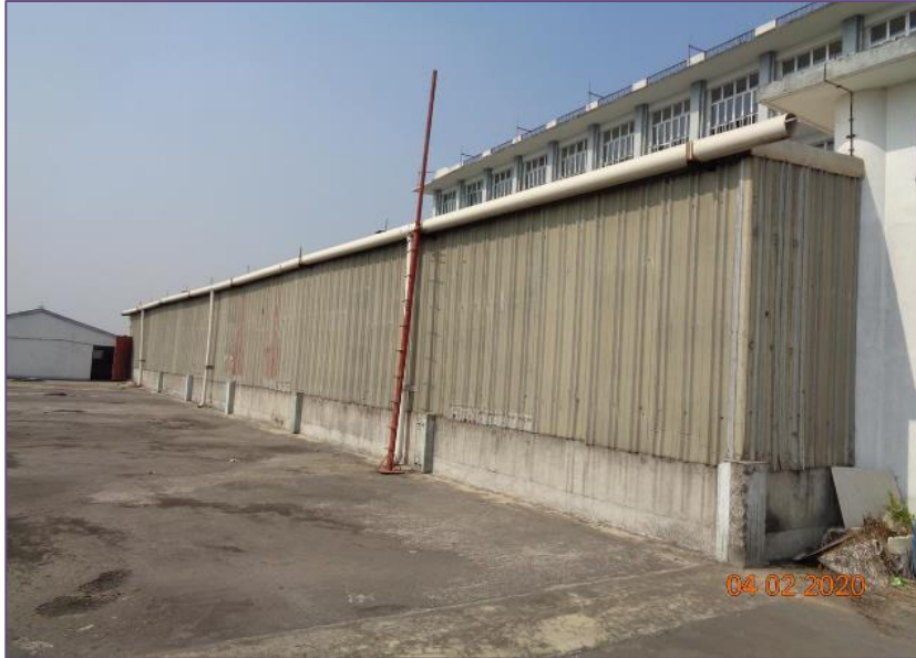
Steel shed at roof
