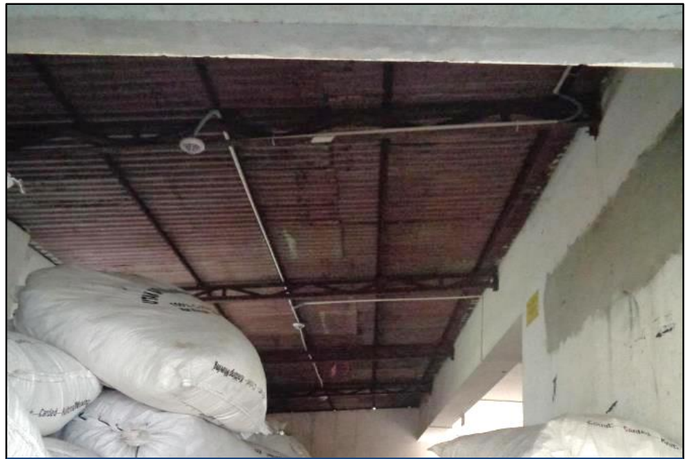
Trusses are connected to the beam of main building
