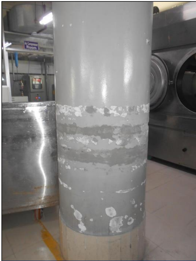
Washing Extension Building
