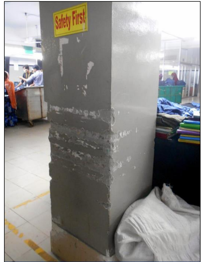
Thermo Oil Building
