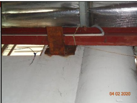
Connections of steel sheds
