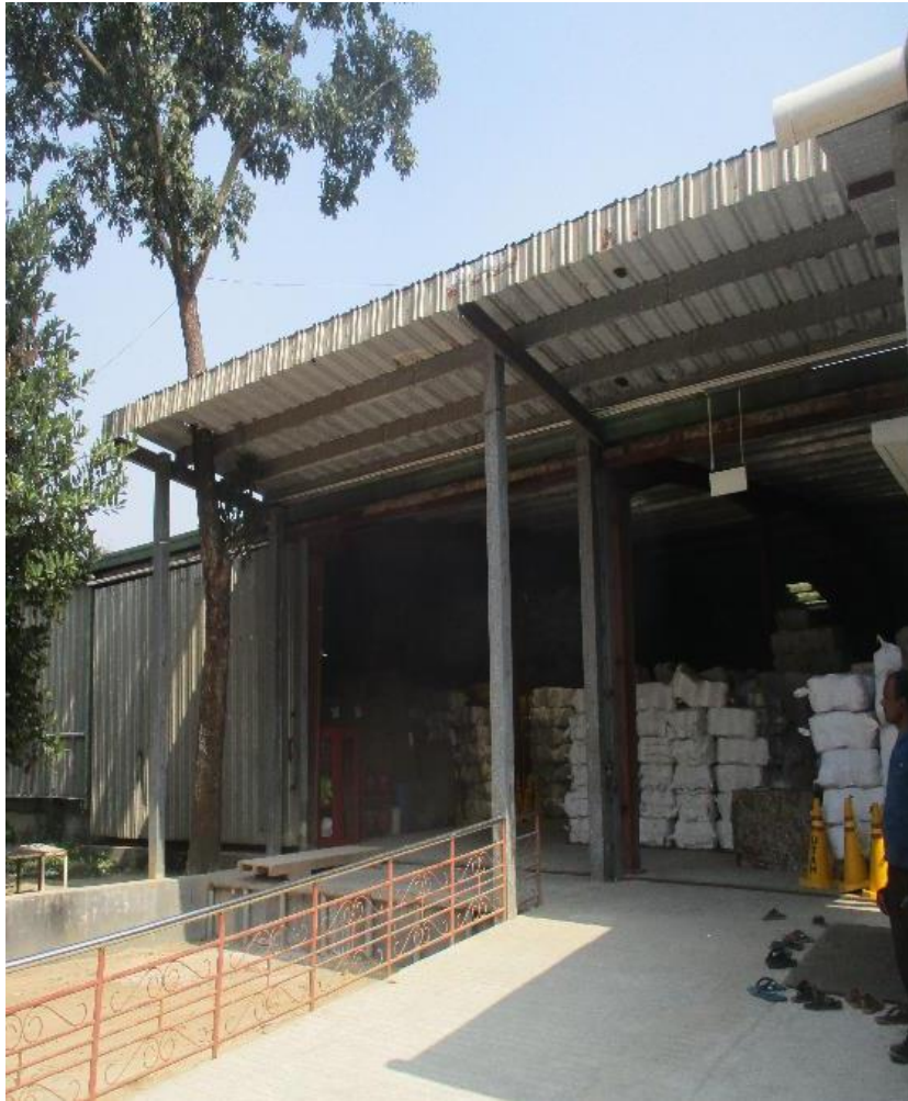
Canopy at front side of the shed
