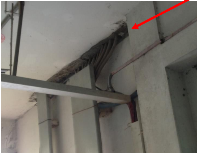
Holes through slabs and beams
