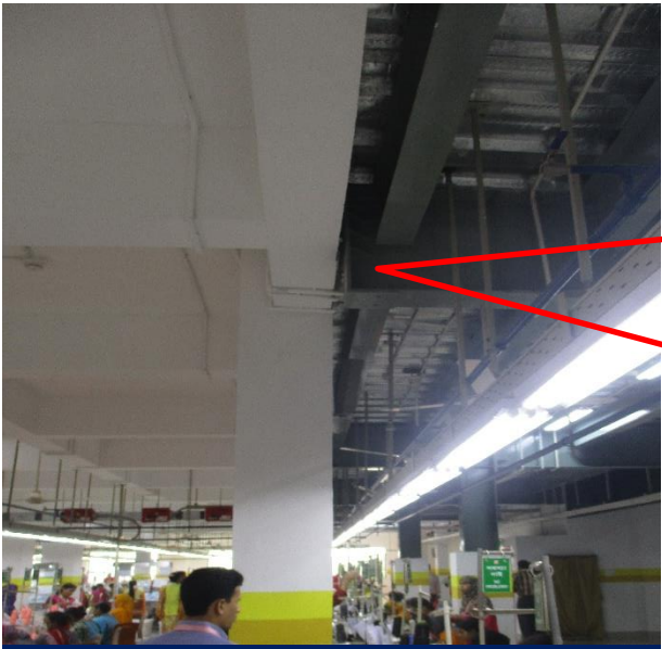
Bolted connection between RC column and steel beam
