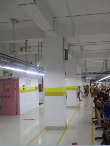
Newly constructed column
