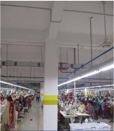
Three side retrofitted column on movement joint
