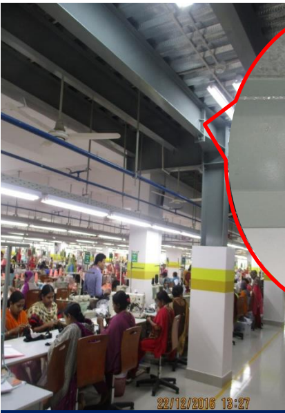
Loose connection observed at beam joint on several area
