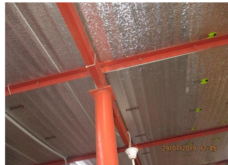
Connection between frame and column
