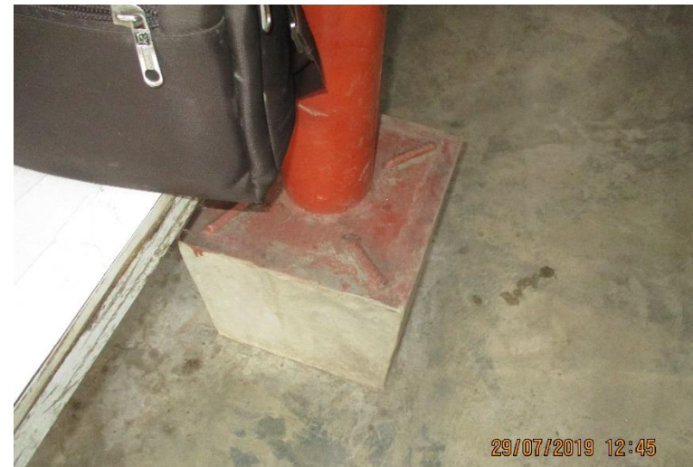
Connection between M/S column and pedestal column
