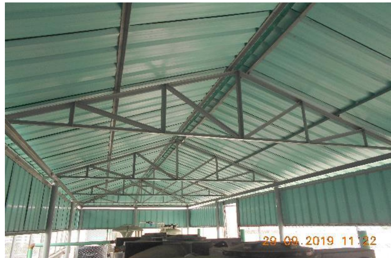
Truss system of the roof shed.
