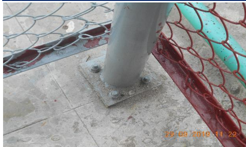
Column base connection .
