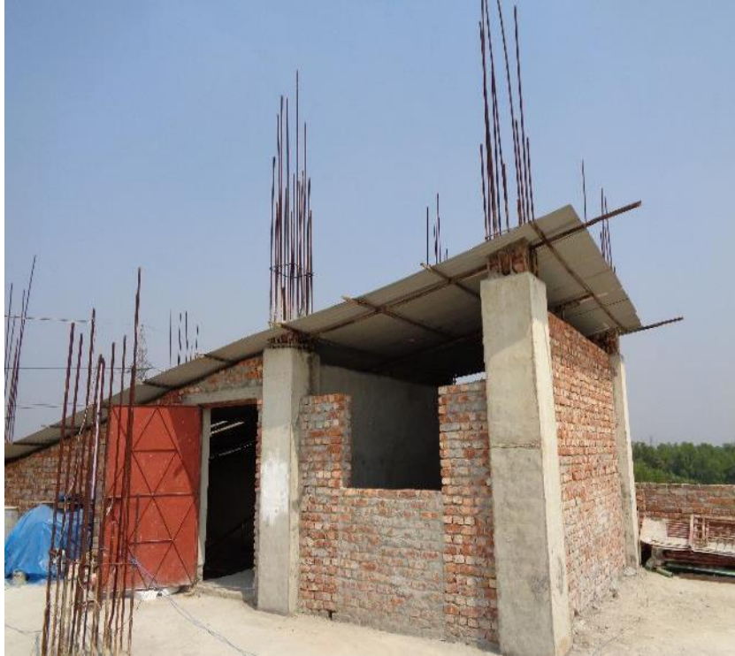
Non engineer steel roof at north stair
