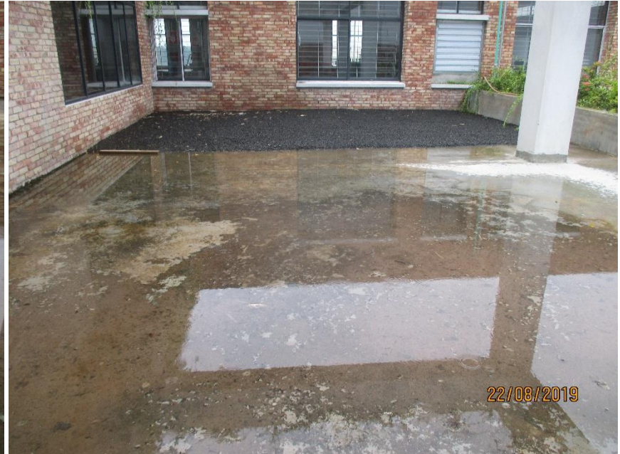
Ongoing water proofing work
