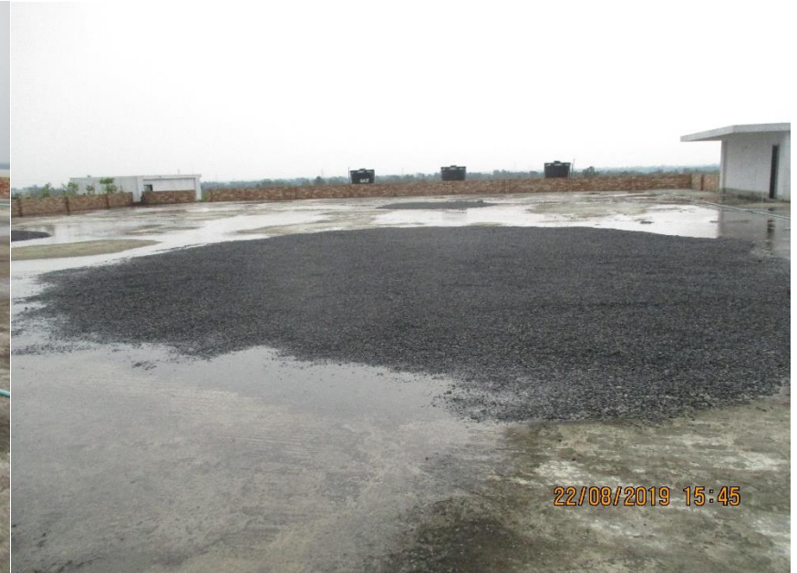
Ongoing water proofing work
