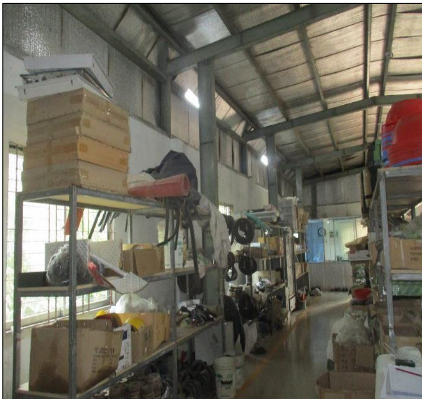
Roof bracing provided along short direction
