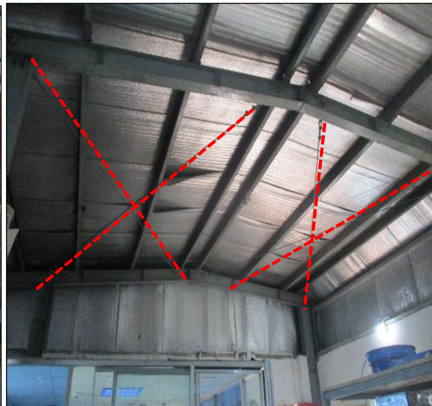
Roof bracing provided along short direction
