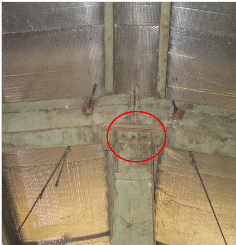
Bolts were missing at several locations
