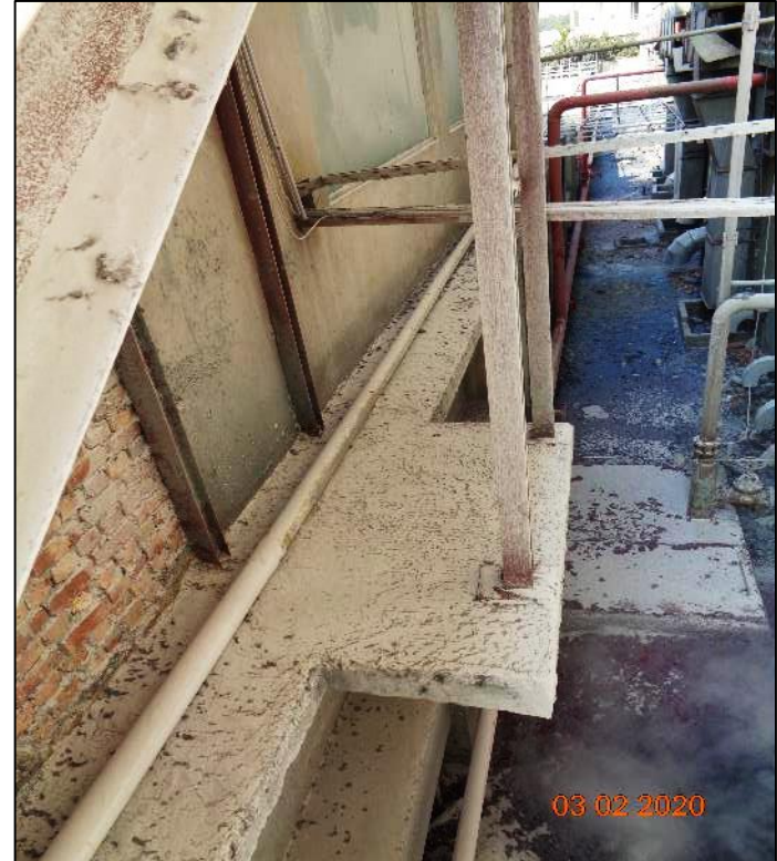
Pier resting on cantilever slab
