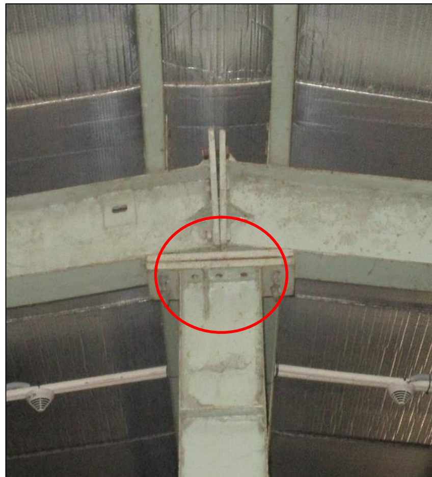
Bolts were missing at several locations
