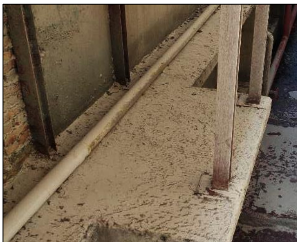
Connection of steel stair
