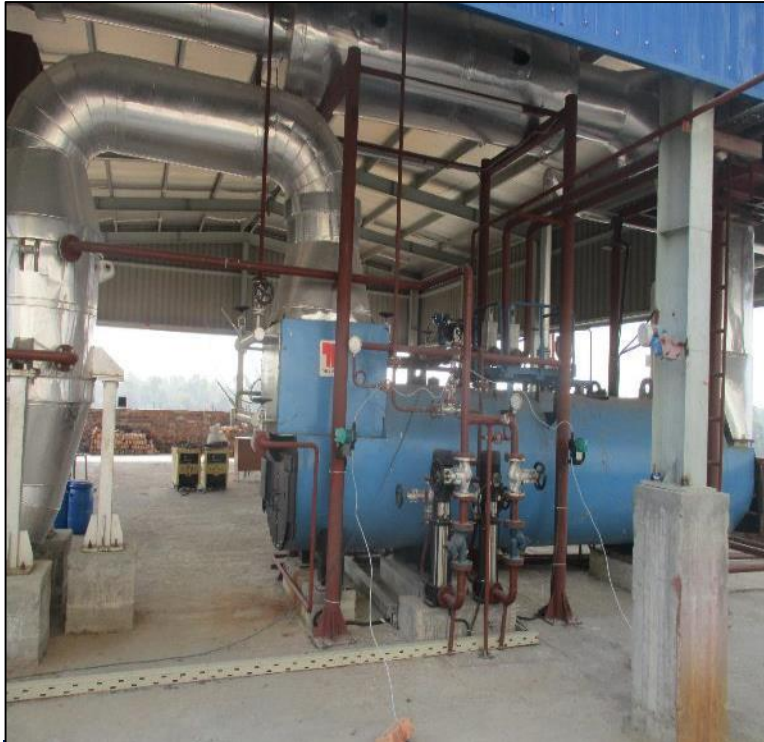
Heavy Boiler machine placed on roof slab
