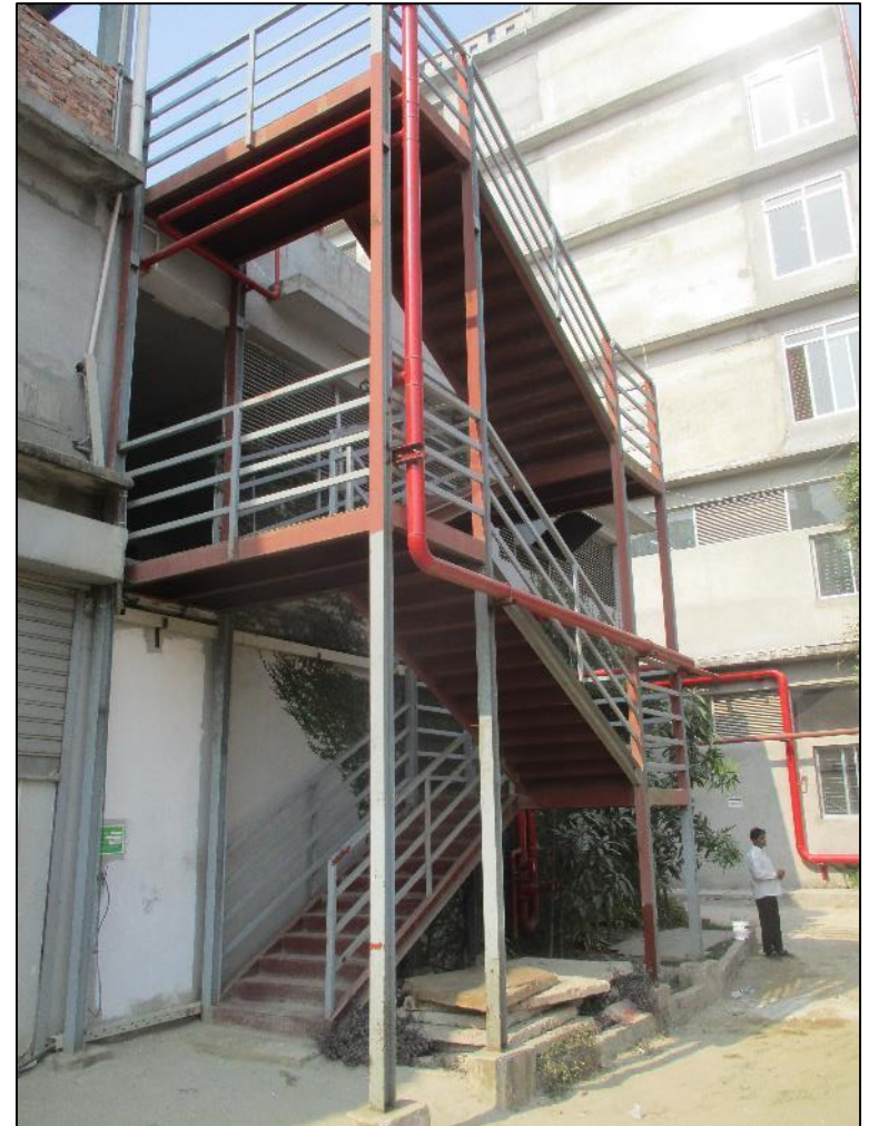
Apparently inadequate steel member size and no stability system provided.
