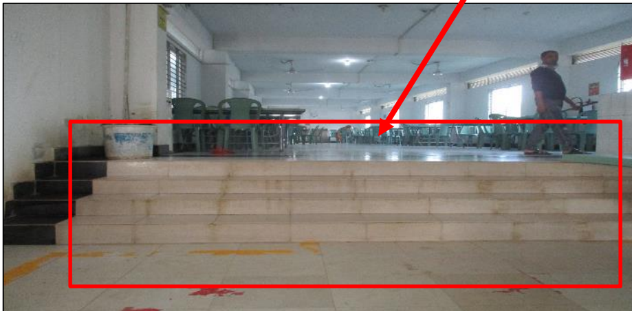
Expansion joint filled with rigid material
