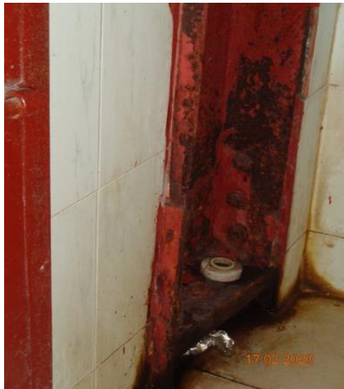
Corrosion in steel column at toilet Zone.
