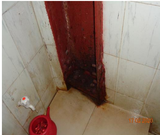
Corrosion in steel column at toilet Zone.
