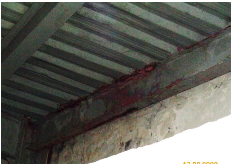
Corrosion in steel beam at toilet Zone.
