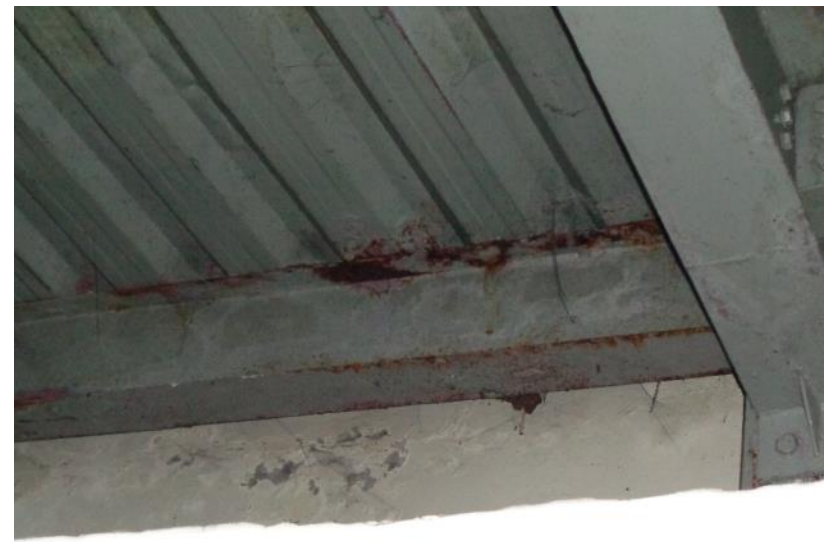
Corrosion in steel beam at toilet Zone.
