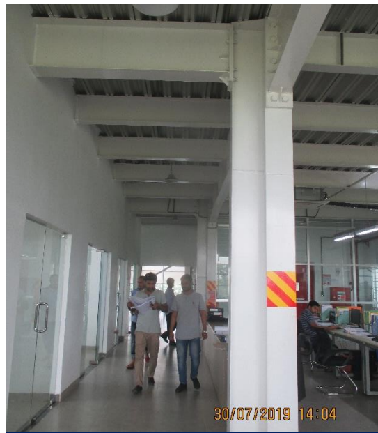
Portal Bracing on 1 st floor
