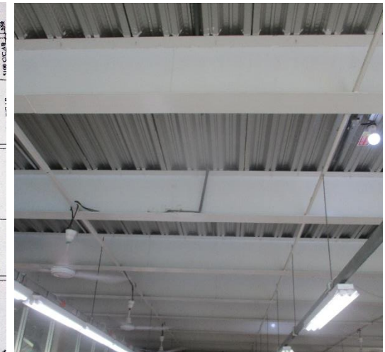
Joist on 1 st floor
