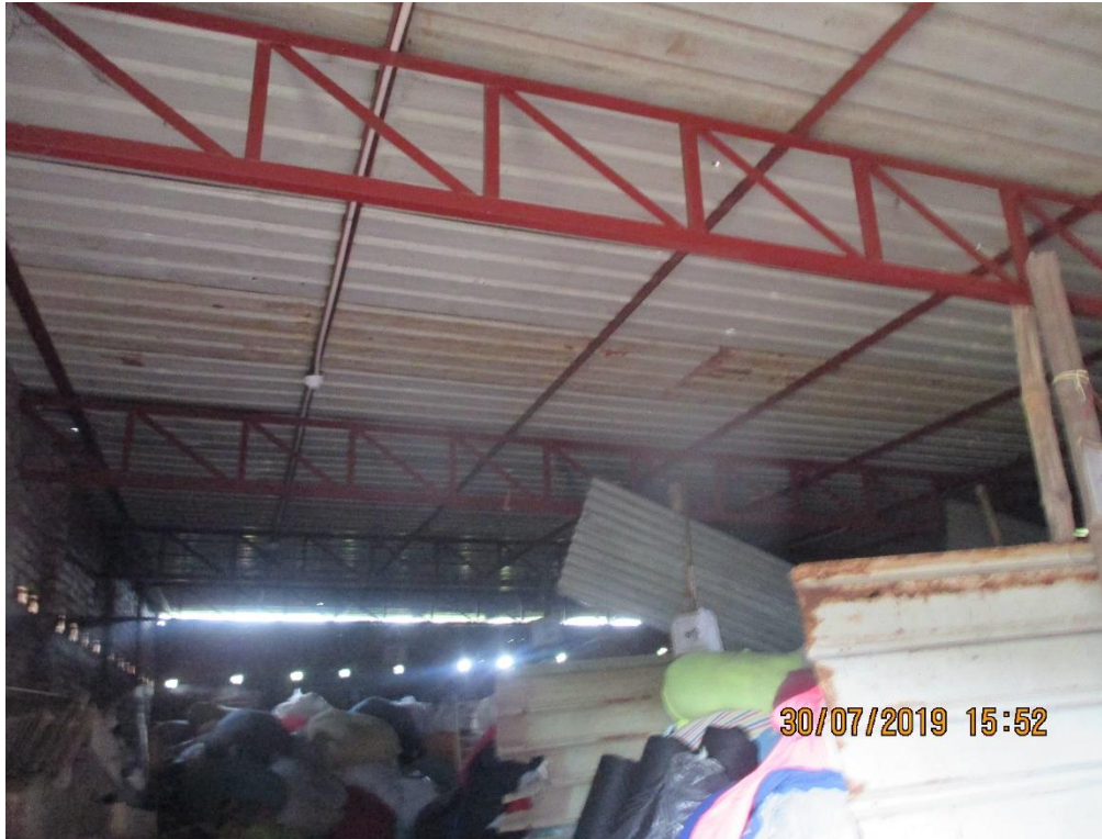
Light weight roof supported on peripheral wall
