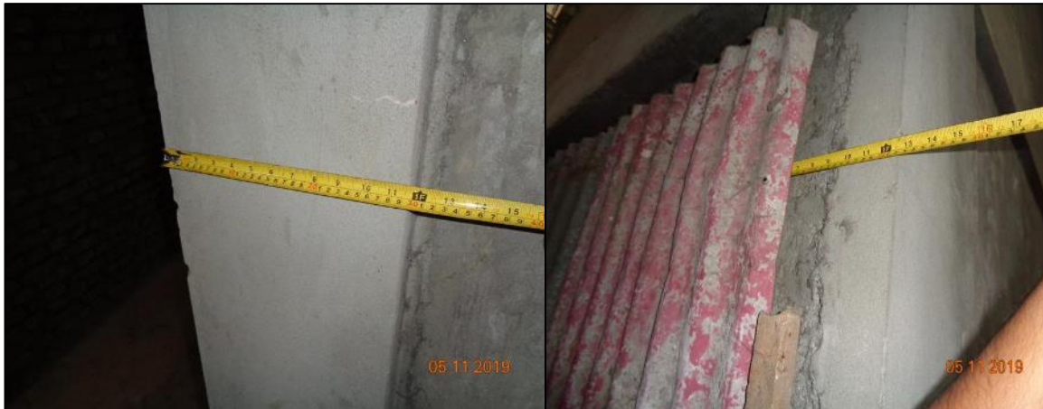
Column size was found 300mmX250mm
