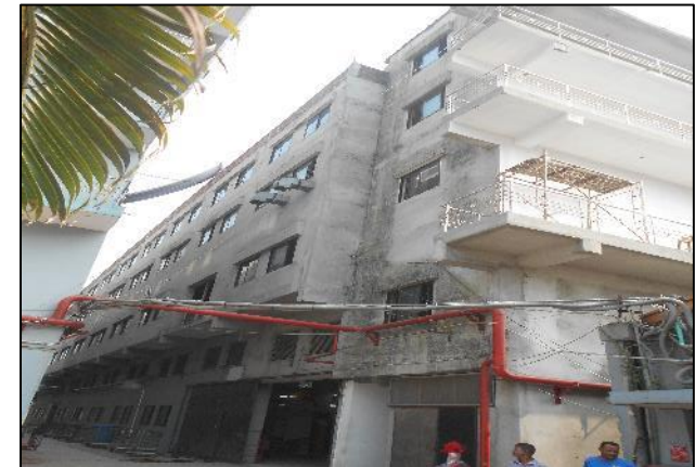
Existing four Storied Building
