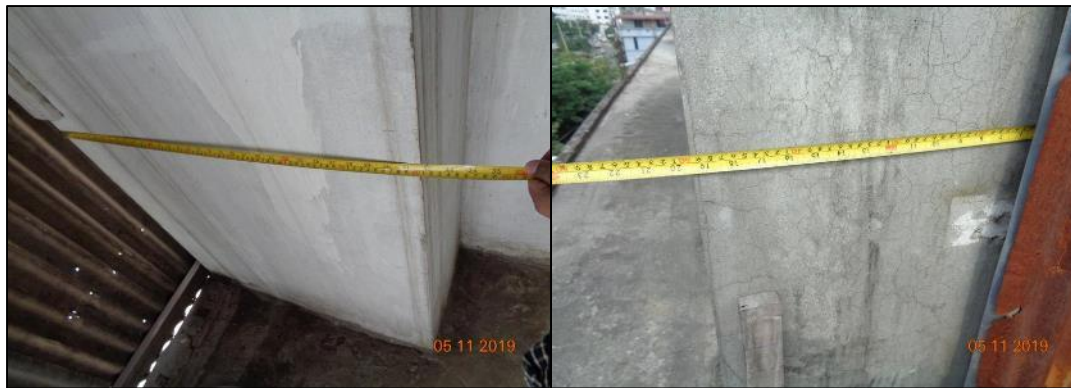
Actual Size of column was found 750mmX450mm
