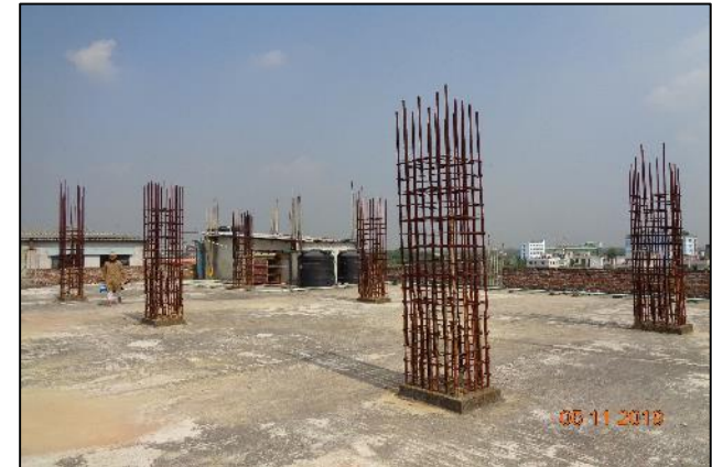
Rebar extension at roof level
