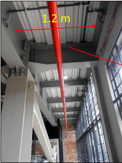
Cantilever portion was observed in the north side from 2 nd floor to 4 th floor
