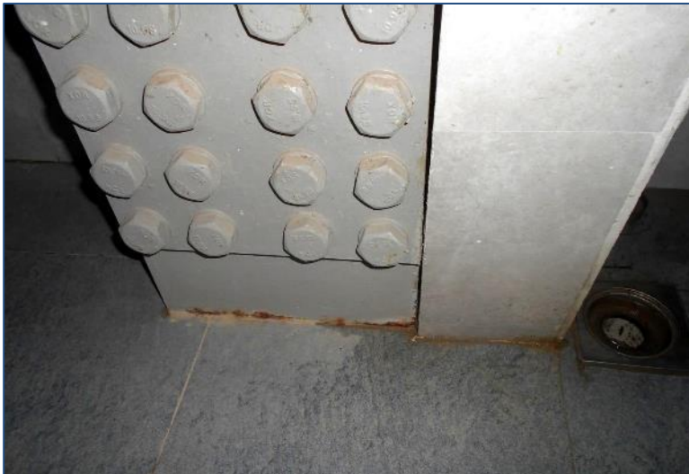
Corrosion found in column and bracing joint connection.
