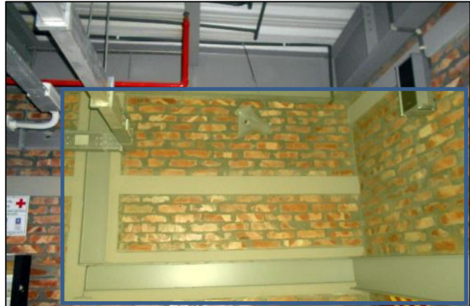
Stair landing supporting system from main beam
