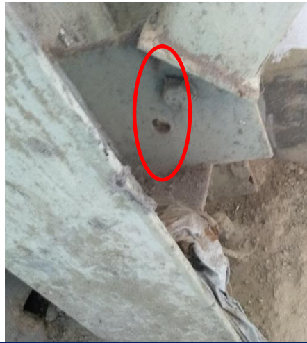
Bolt missing at bracing connection
