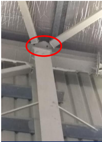
Bolt missing at bracing connection
