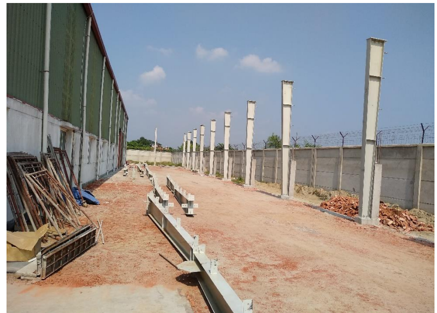
Additional Steel column
