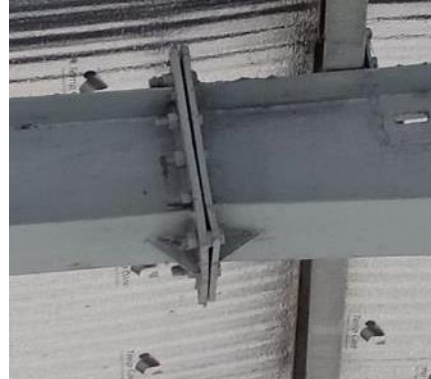
Gap in between beam-column joint
