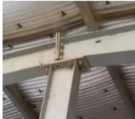
Bolt missing in connection
