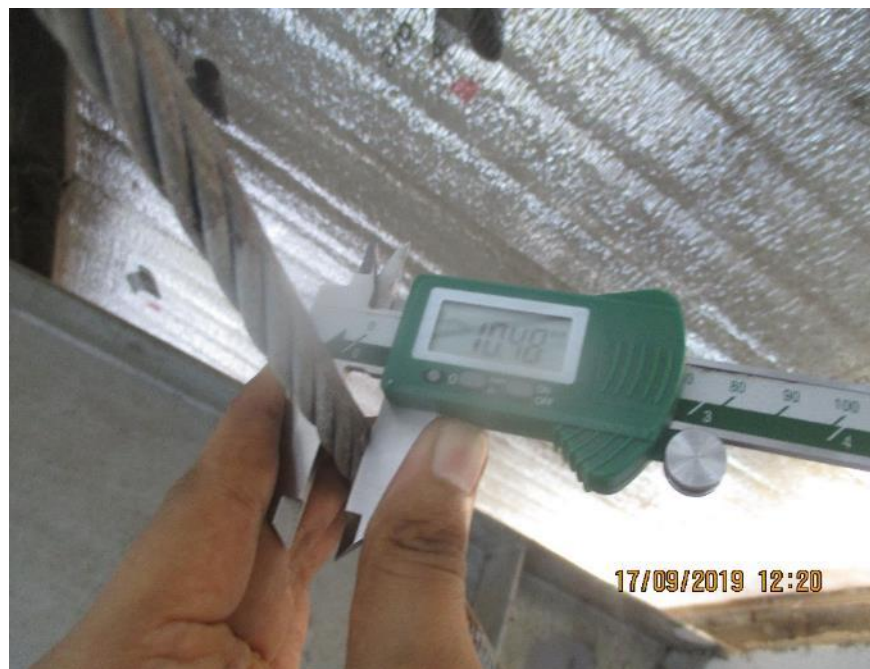
10 mm roof cable bracing
