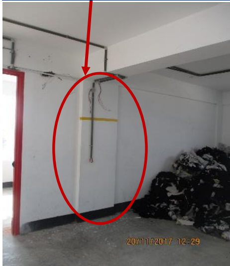
Marked Columns size found 300mm x 680mm which are denoted as C2 (300mm x 500mm) type column in column layout
