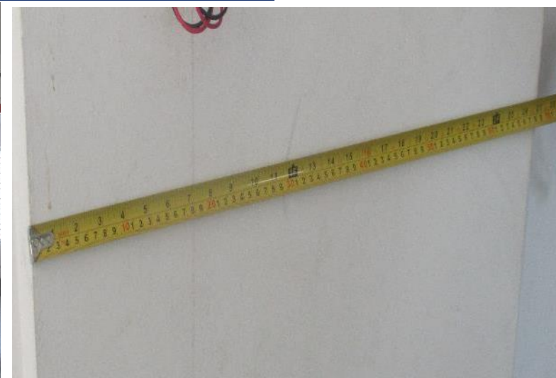
Marked column size in long direction was measured 680mm
