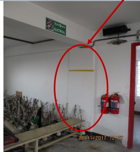
Marked Columns size found 300mm x 680mm which are denoted as C2 (300mm x 500mm) type column in column layout
