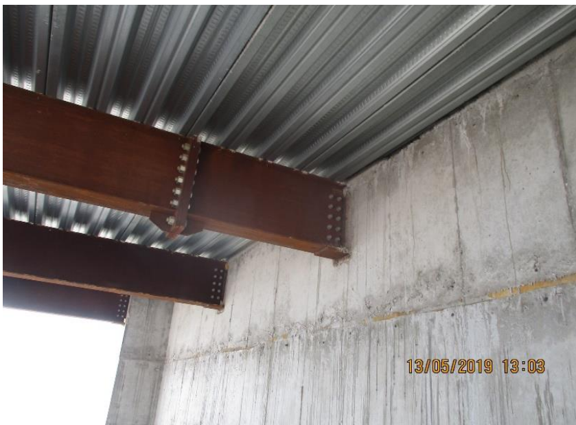
Connection between steel beam and shear wall
