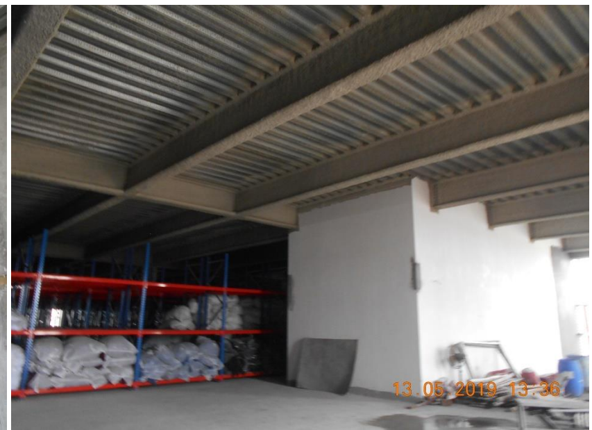
Connection between steel beam and shear wall
