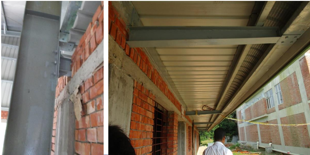
Canopy observed at south
