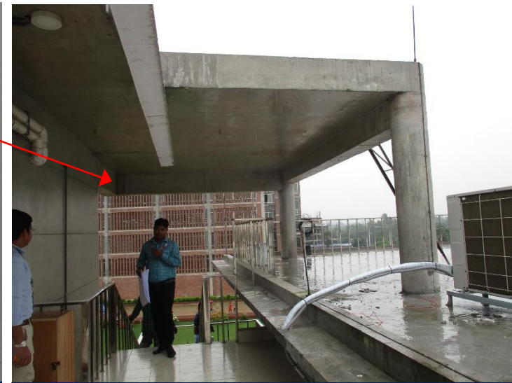
Beam at roof level not match with dwg.
