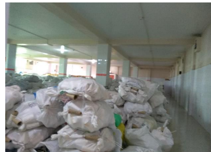
Observed floor loading
