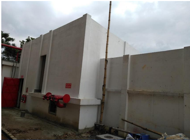
Fire pump room
