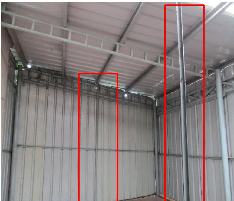
Single angle provide as column
