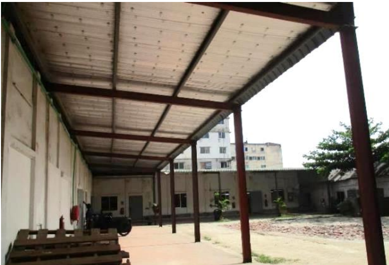
No compression strut and bracing at roof
