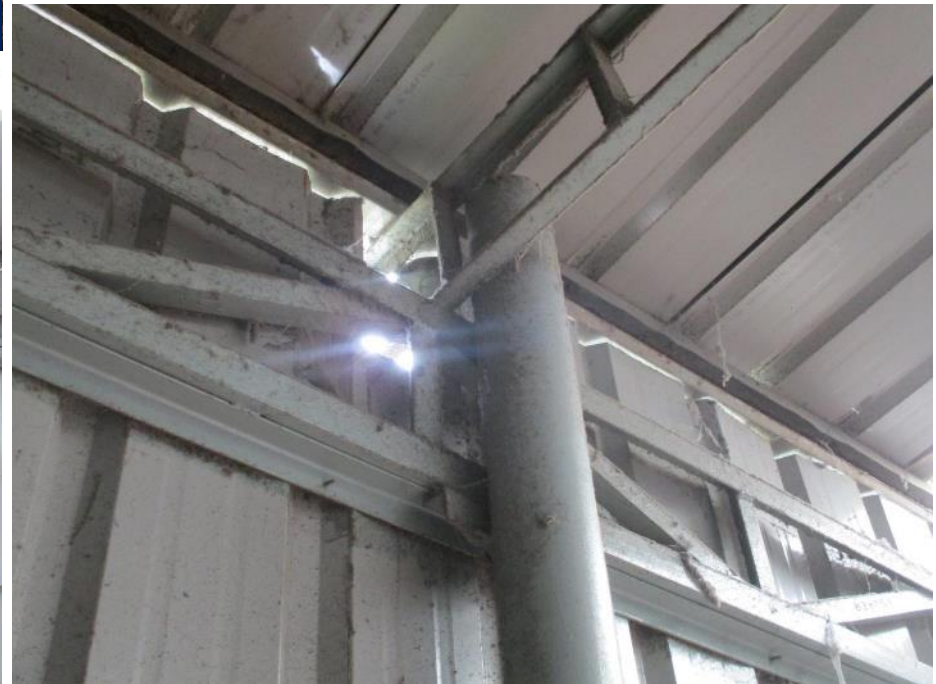
Connection between vertical member and roof truss
