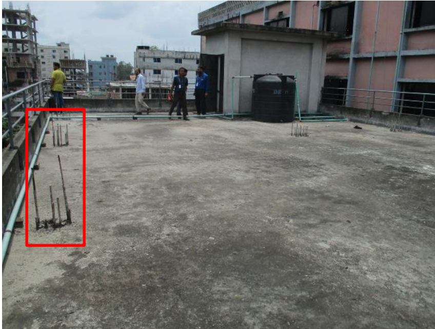
Exposed rebars on roof slab.
