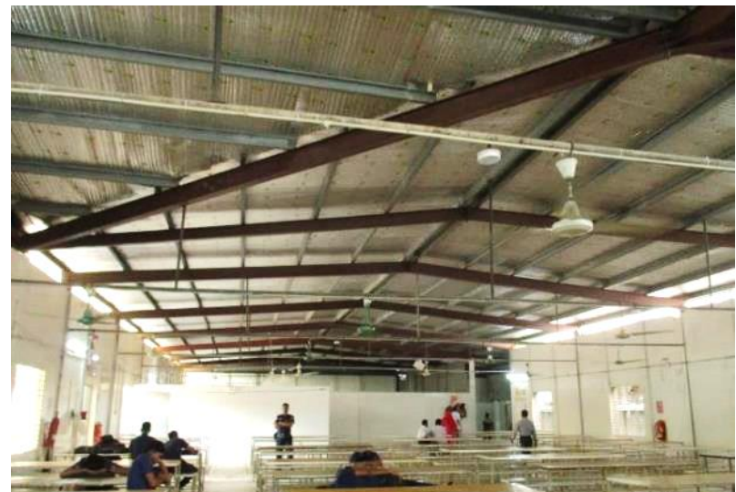
No compression strut and bracing at roof
