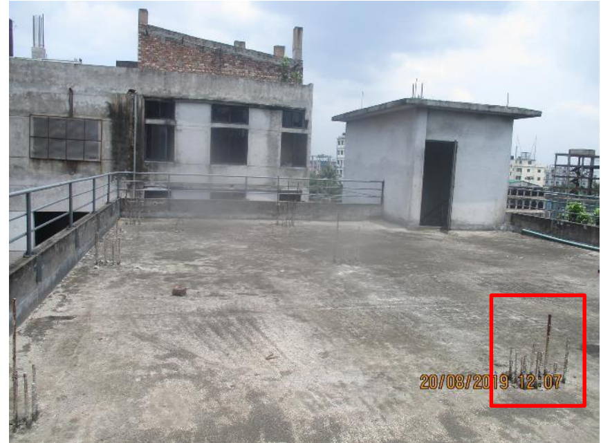
Exposed rebars on roof slab.
