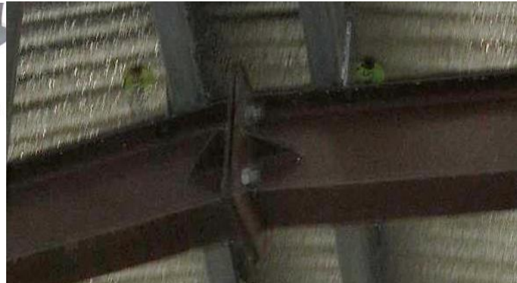
Significant gap between joint plates and support
