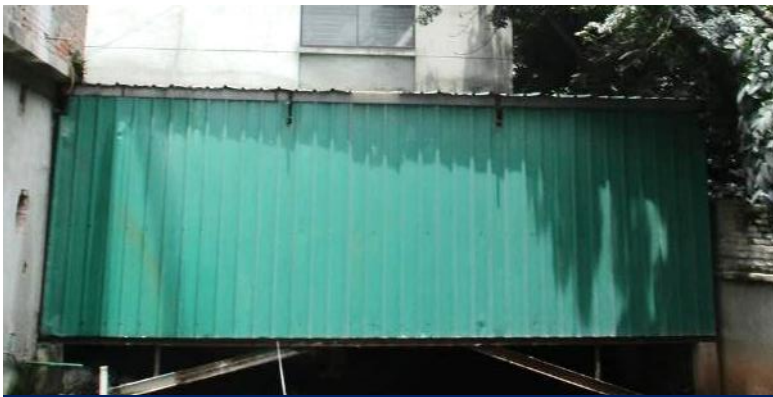
The bottom support system of steel deck
