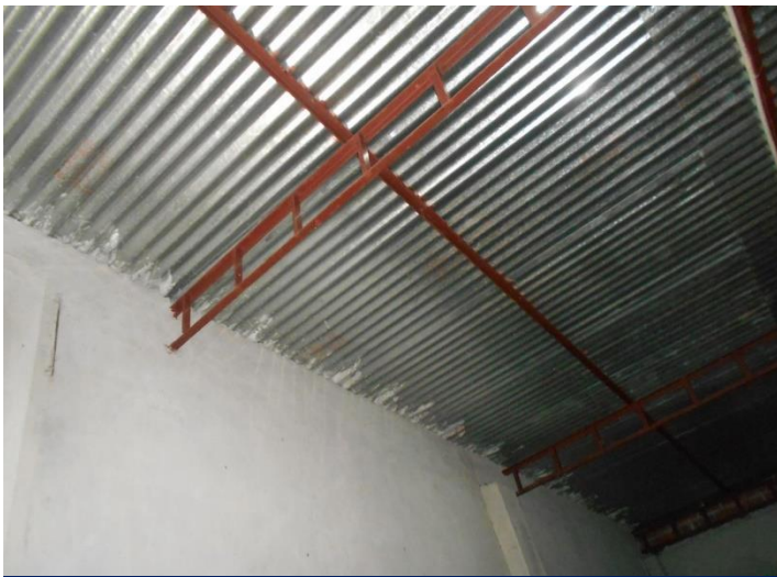
Truss-Brick wall connection
