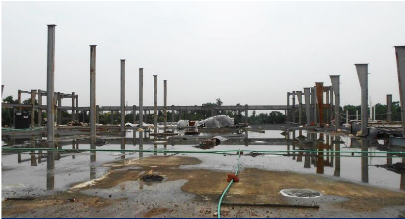
Under construction frame on 3 rd floor
