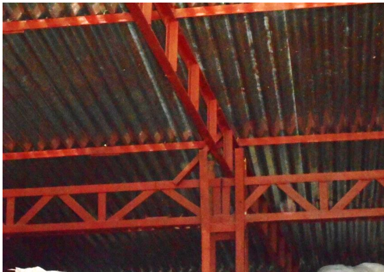
Roof truss system
