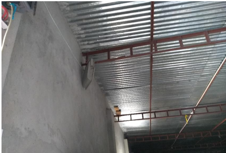
Truss inserted into brick wall
