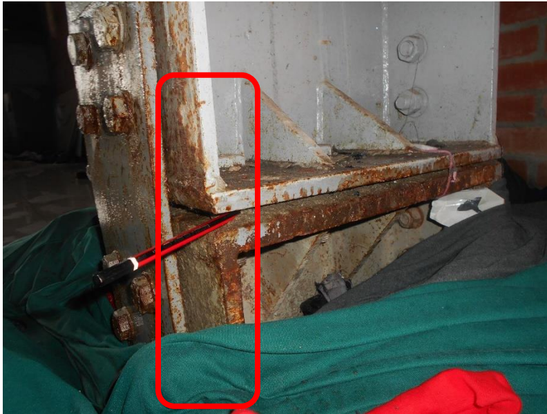
Gap in between beam-column joint
