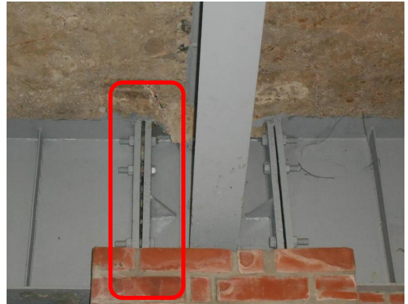
Gap in between beam-column joint
