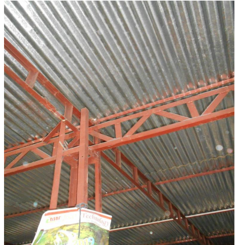
Roof without bracing
