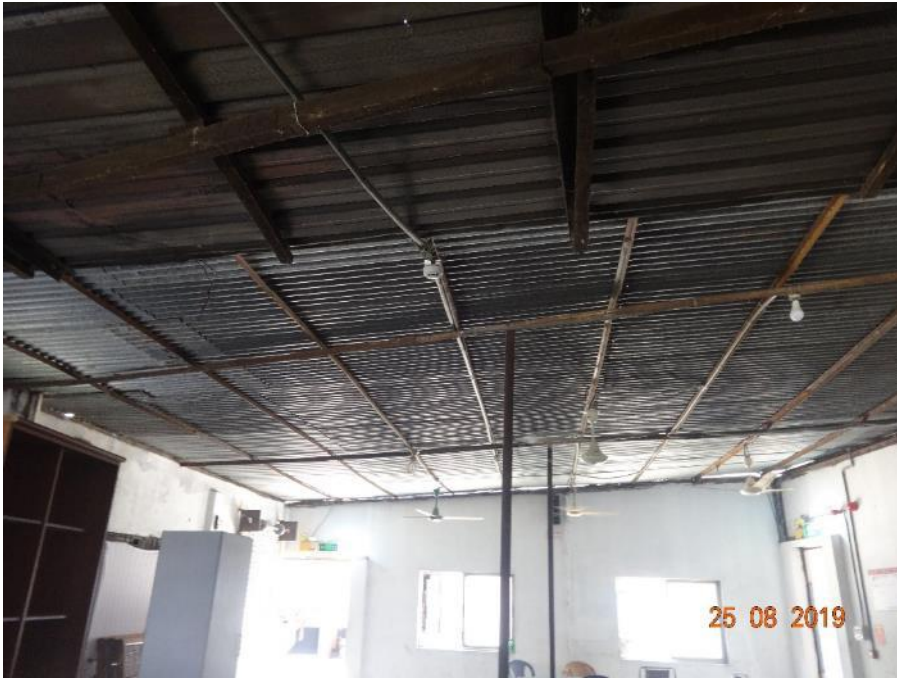
Light weight roof supported on peripheral wall
