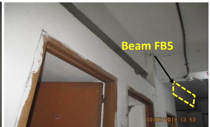
Beam FB5 was found offset towards west from grid I2'.
