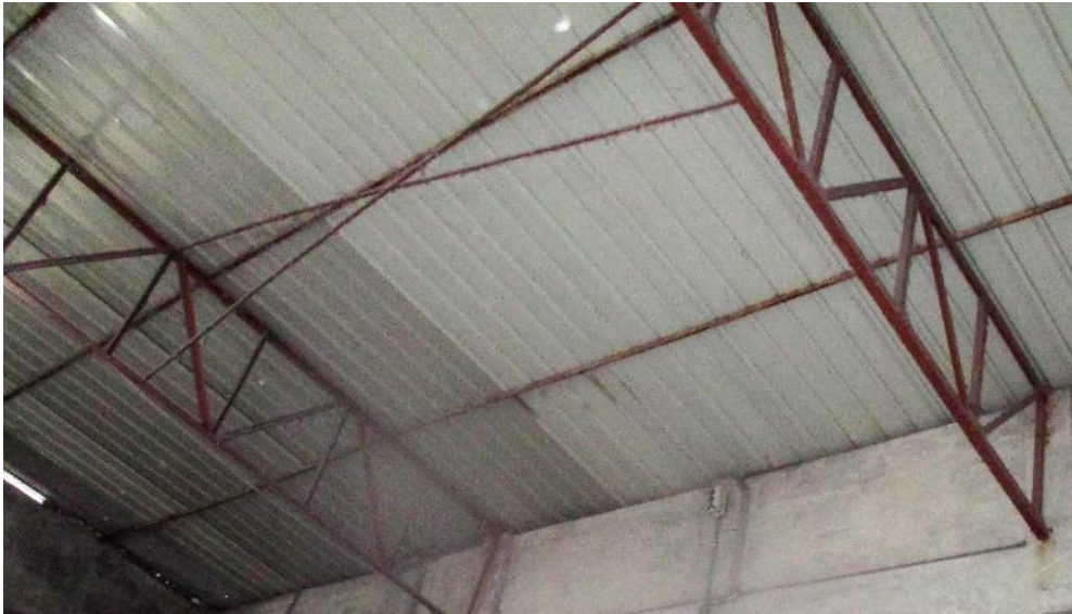
Bracings in old part of the Dyeing Shed
