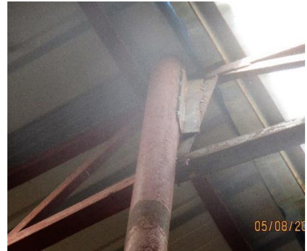
Rafter-column connection
