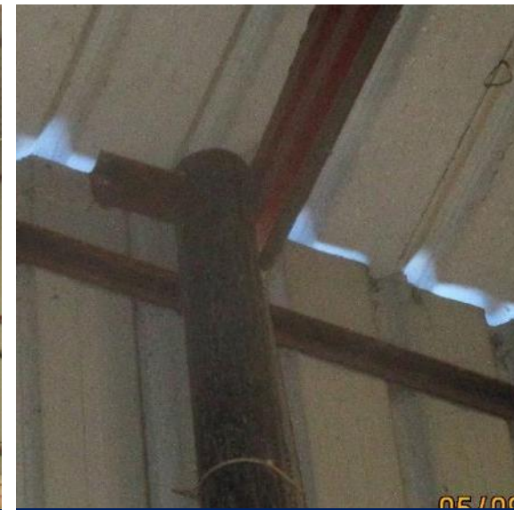
Rafter-column connection
