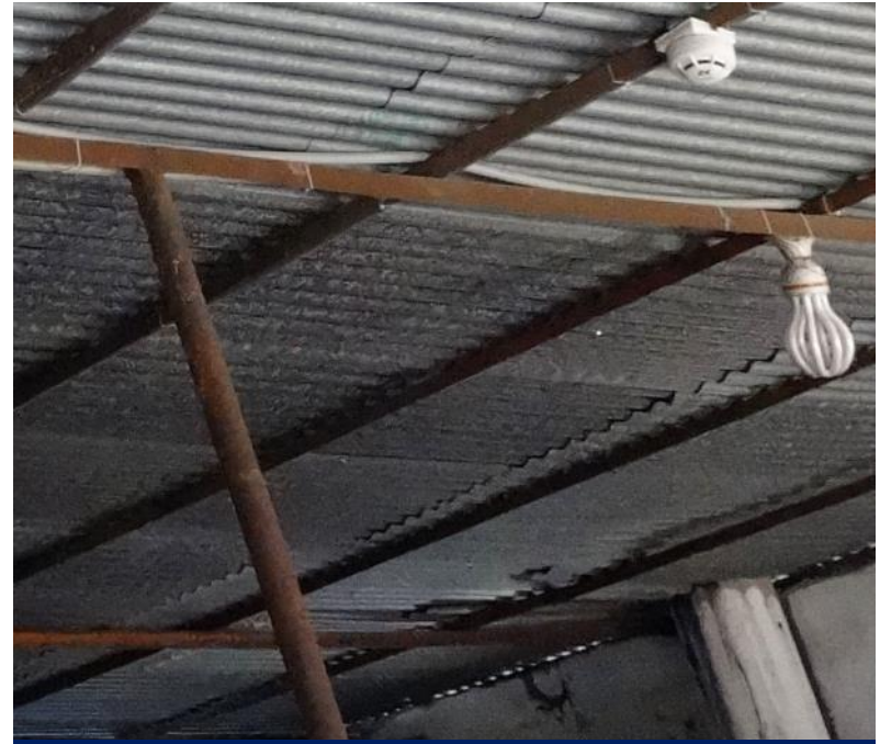
Non-engineered connection
