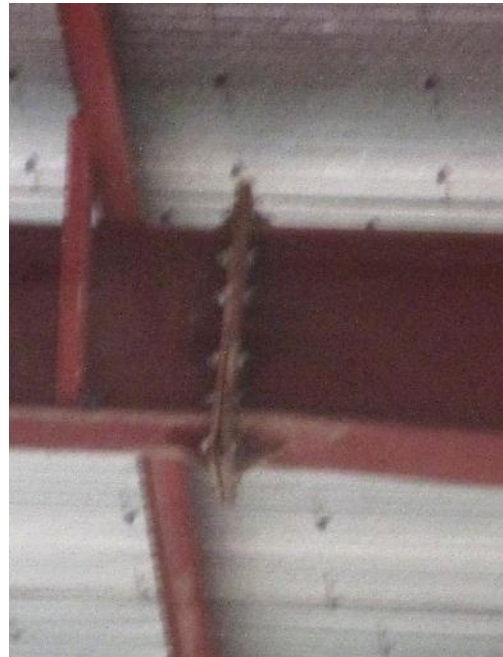
Gap between rafter-rafter connections
