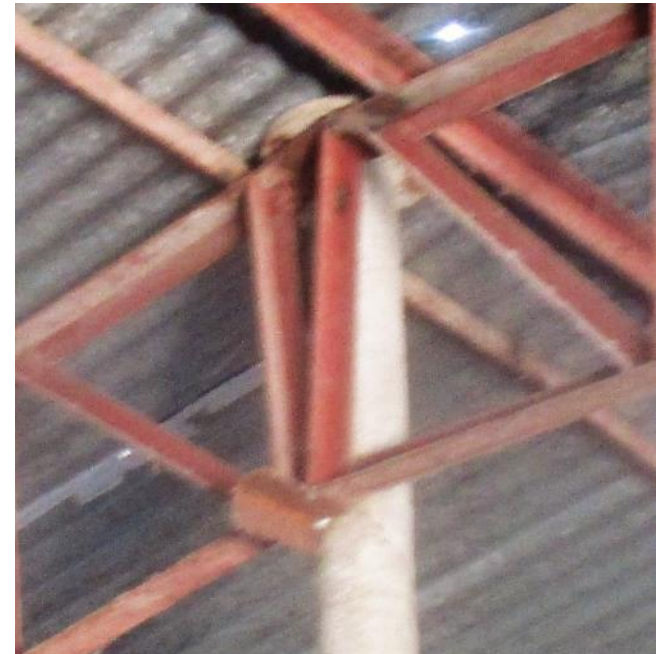
Truss-column connection
