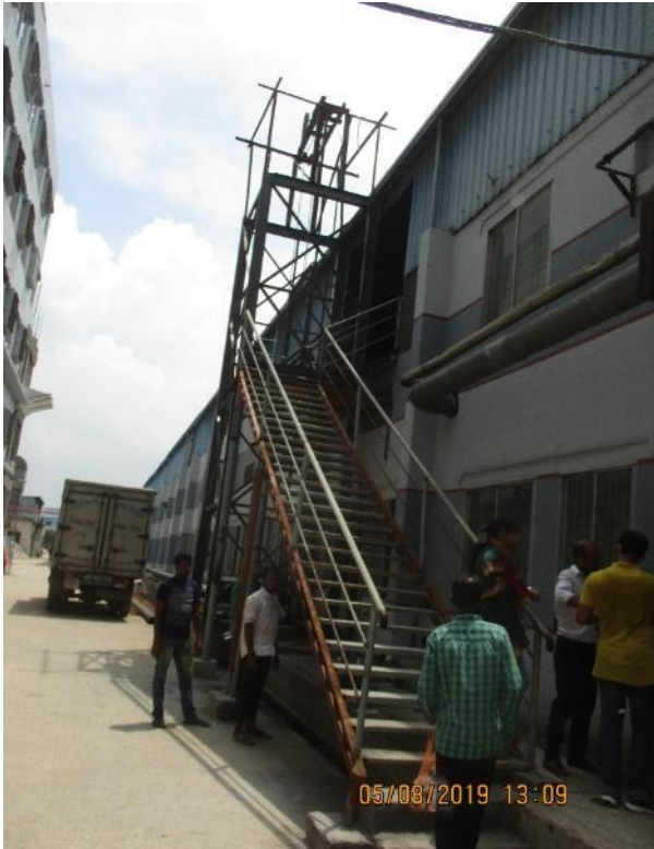
Undocumented steel stair adjacent to dyeing shed
