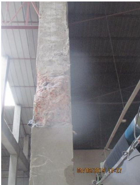
Beams were cut off at some locations.
