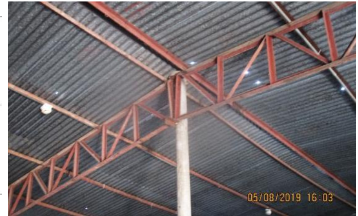
Truss framing in the shed
