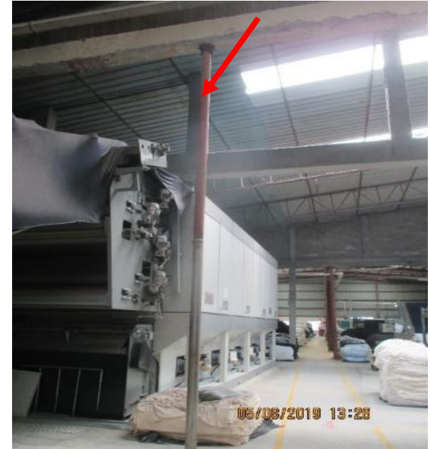
Two RC columns were replaced by a steel pipe
