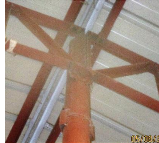
Rafter-column connection
