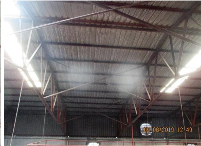
Bracings in old part of the Dyeing Shed
