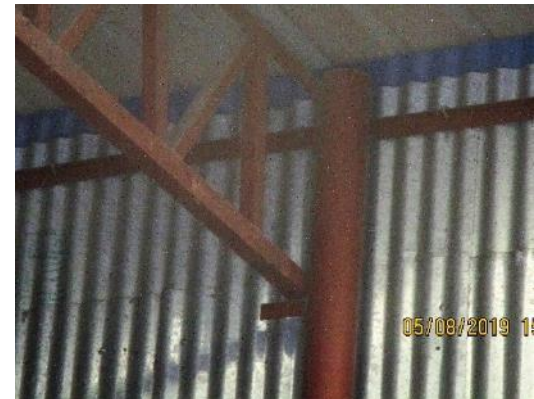
Rafter-column connection
