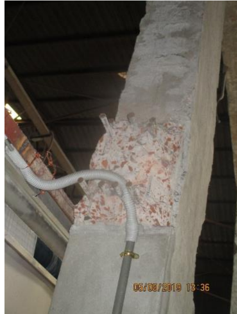
Beams were cut off at some locations.
