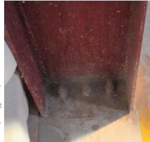
Anchor bolts were 20 mm instead of 25 mm.
