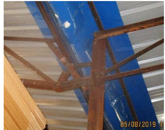
Rafter-column connection
