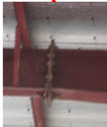
Column-rafters joint has 16-16 mm bolts and rafter-rafters joint has 12-16 mm bolts instead of 16-20 mm bolts as mentioned in as-built drawings.
