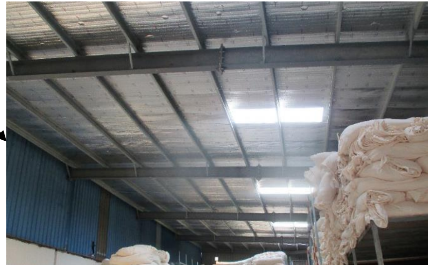
No roof bracing was observed in this part
