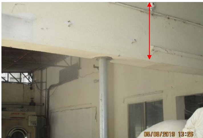
125mm thick and approximately 2m wall
