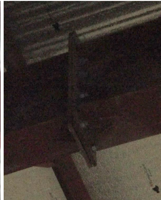
Gap between rafter-rafter connections
