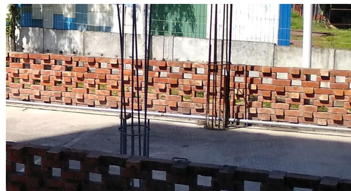
Rebar extension at roof level
