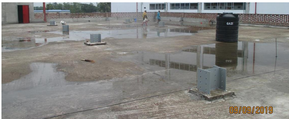
Steel column extension at roof level
