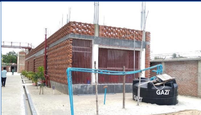
Existing One Storied Building
