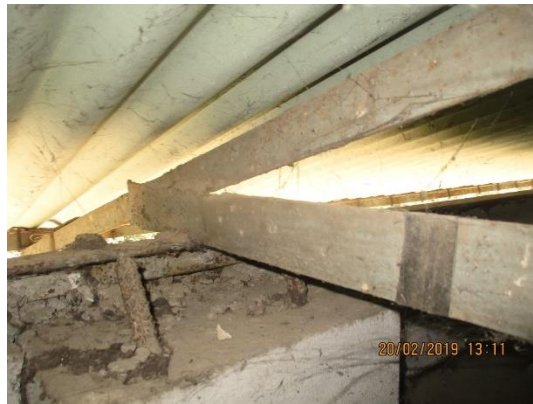
End support condition of truss
