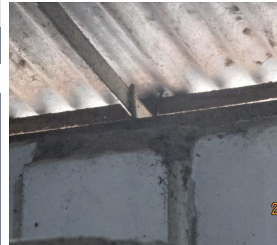
Welded connection between steel member and column's rebar
