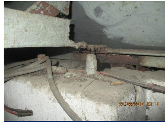
Middle support condition of truss
