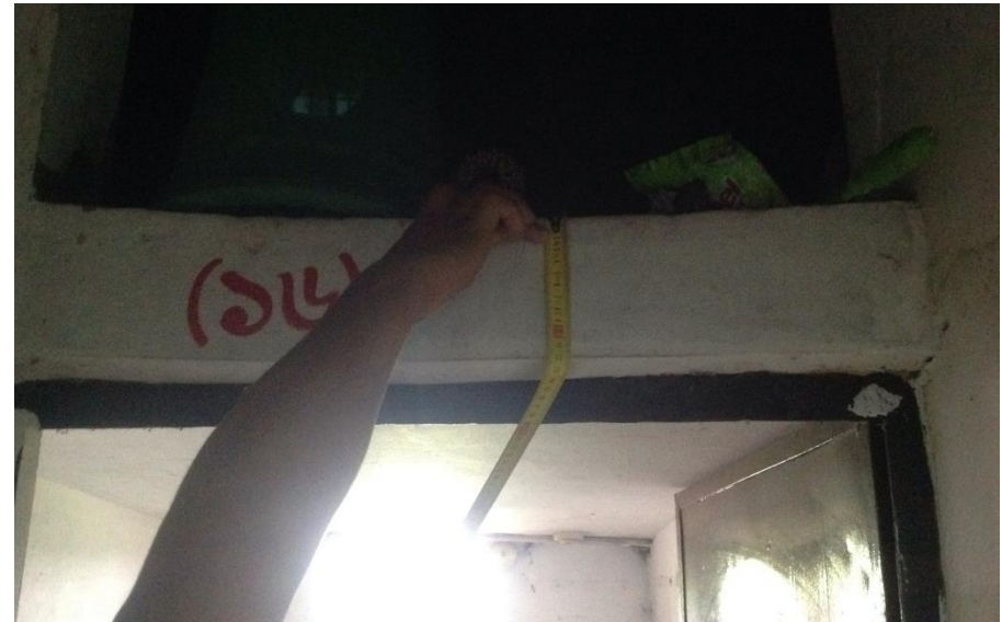
120mm Suspended slab to 1 st Floor Toilet
