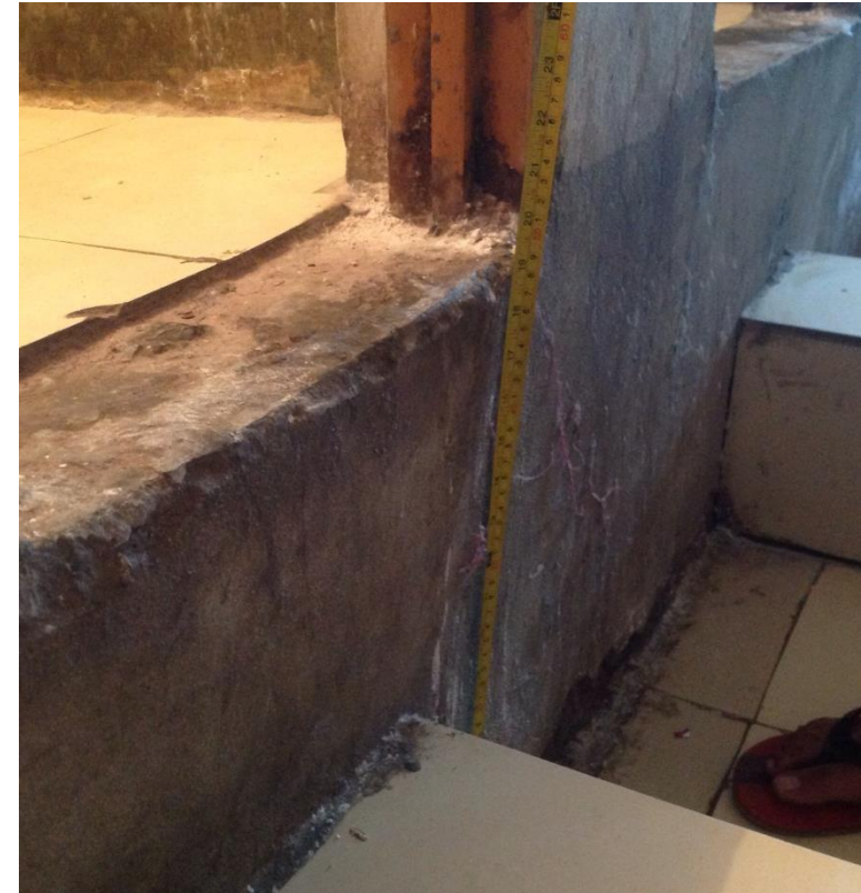
500mm Toilet Plinth to 3 rd Floor
