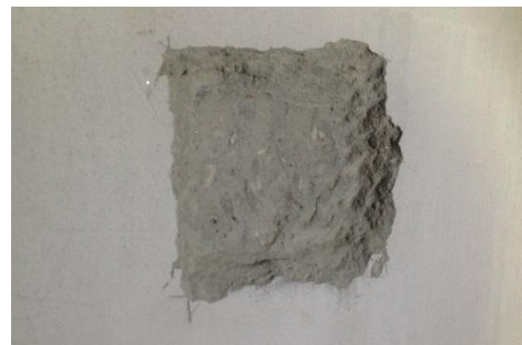
Tested Column D/5 (Stone)
