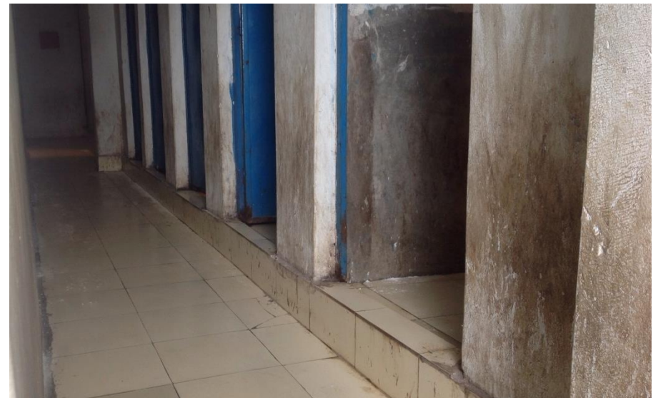
150mm plinths, slabs and walls to 4 th and 5 th Floors
