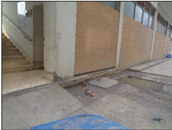
Discontinuous strap footing above ground.
