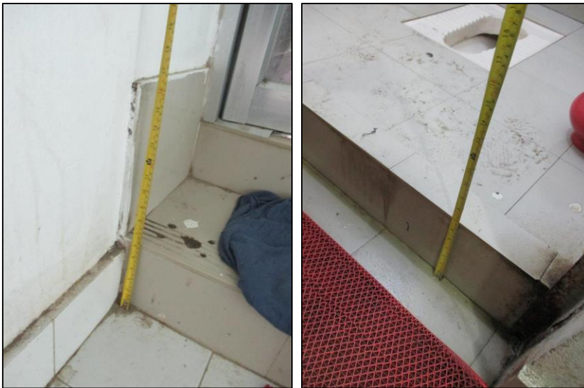
Toilet floor build up
