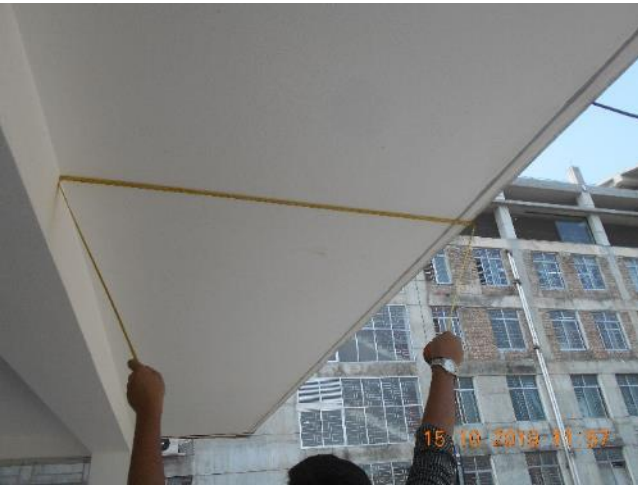
1.21m cantilever at stair top
