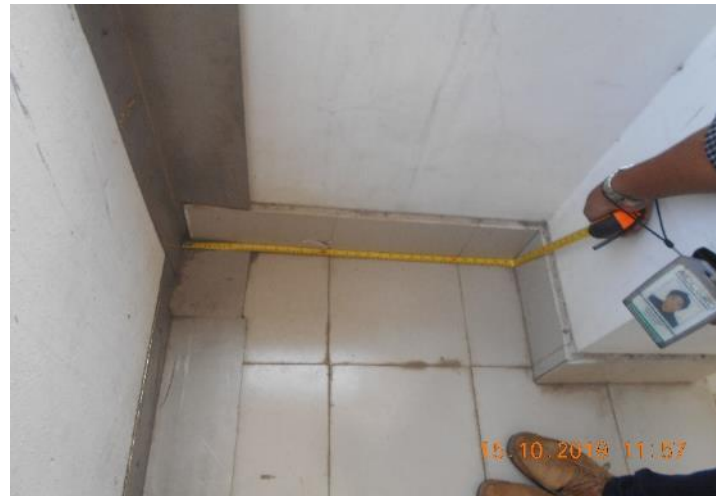
0.8m cantilever at floor level
