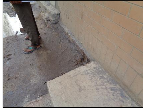
Discontinuous strap footing above ground.
