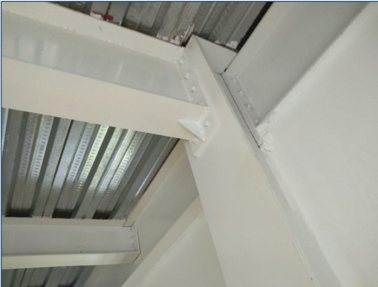
Beam-column joint at top level
