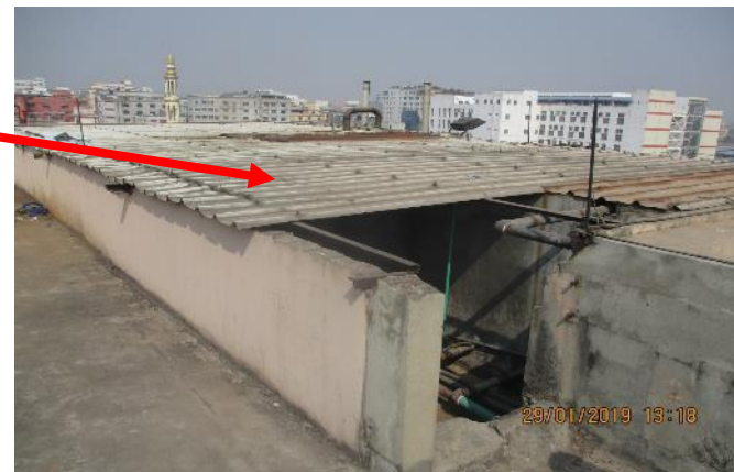
RCC water tank on existing roof
