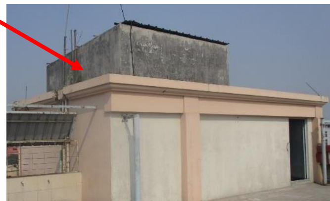
RCC water tank on existing stair case
