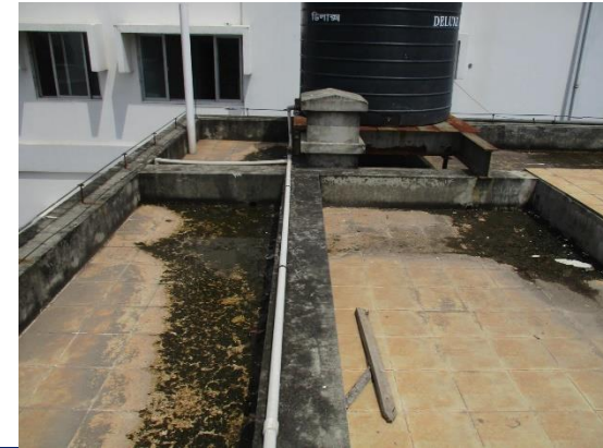
Water ponding was observed on the roof of Medical Building.
