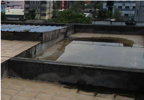
Water ponding was observed on the roof of Medical Building.
