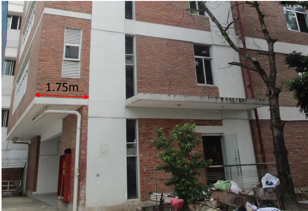
1.75m cantilever slab on north side and 1.33m cantilever slab on east & west side on Medical Building.
