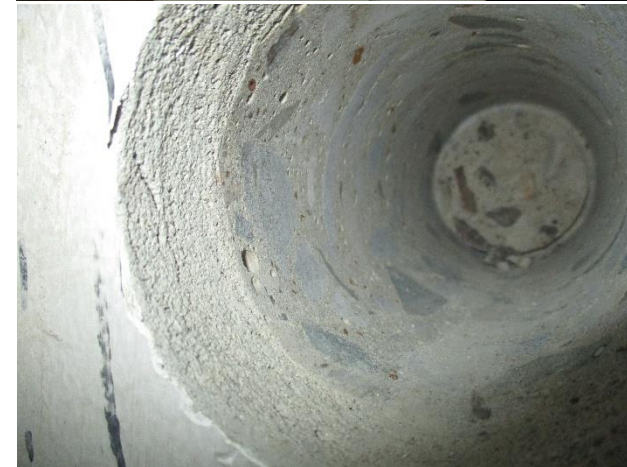
Concrete core cutting from the column of Sub-station Building
