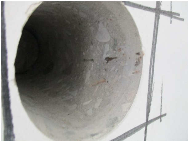
Concrete core cutting from the column of Medical Building
