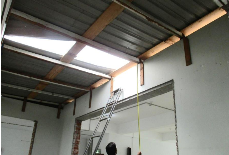
Lightweight roof on Medical Building
