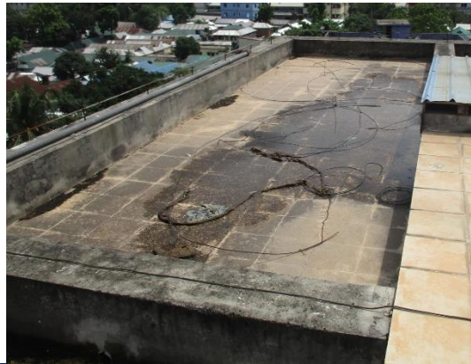
Water ponding was observed on the roof of Medical Building.
