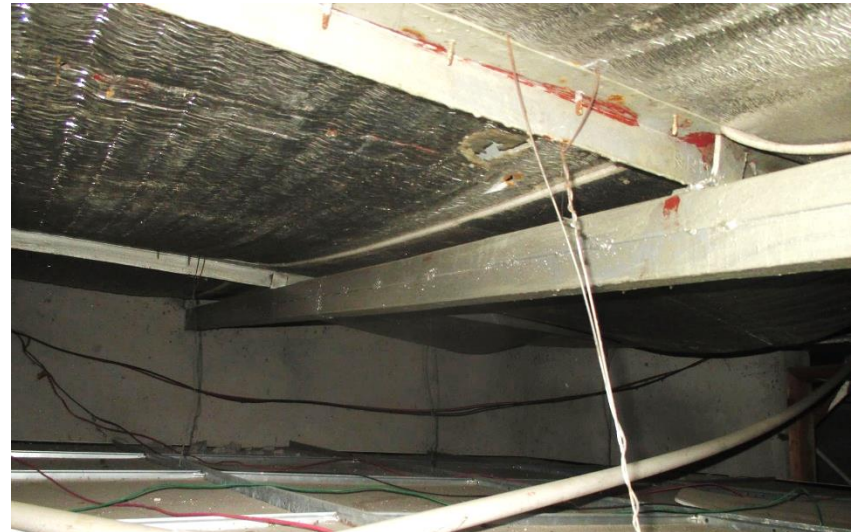
Lightweight roof on Sub-station Building
