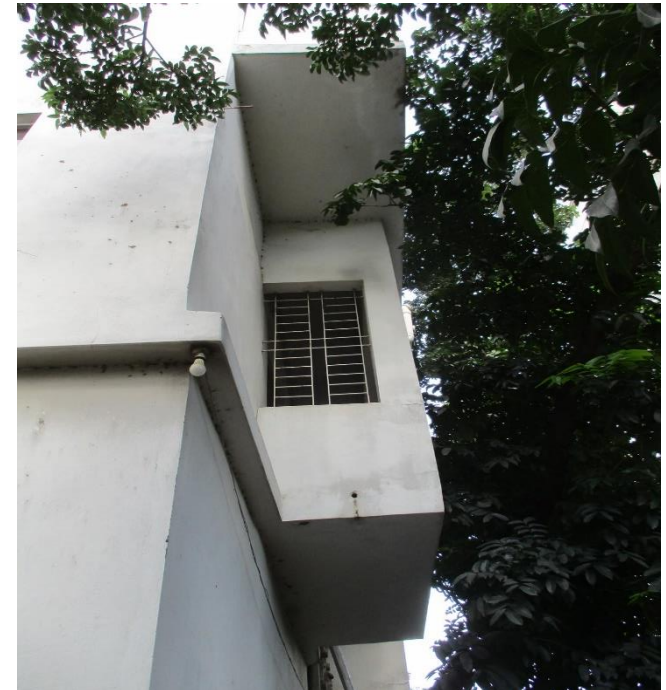
1.2m cantilever slab on south side of Sub-station Building.
