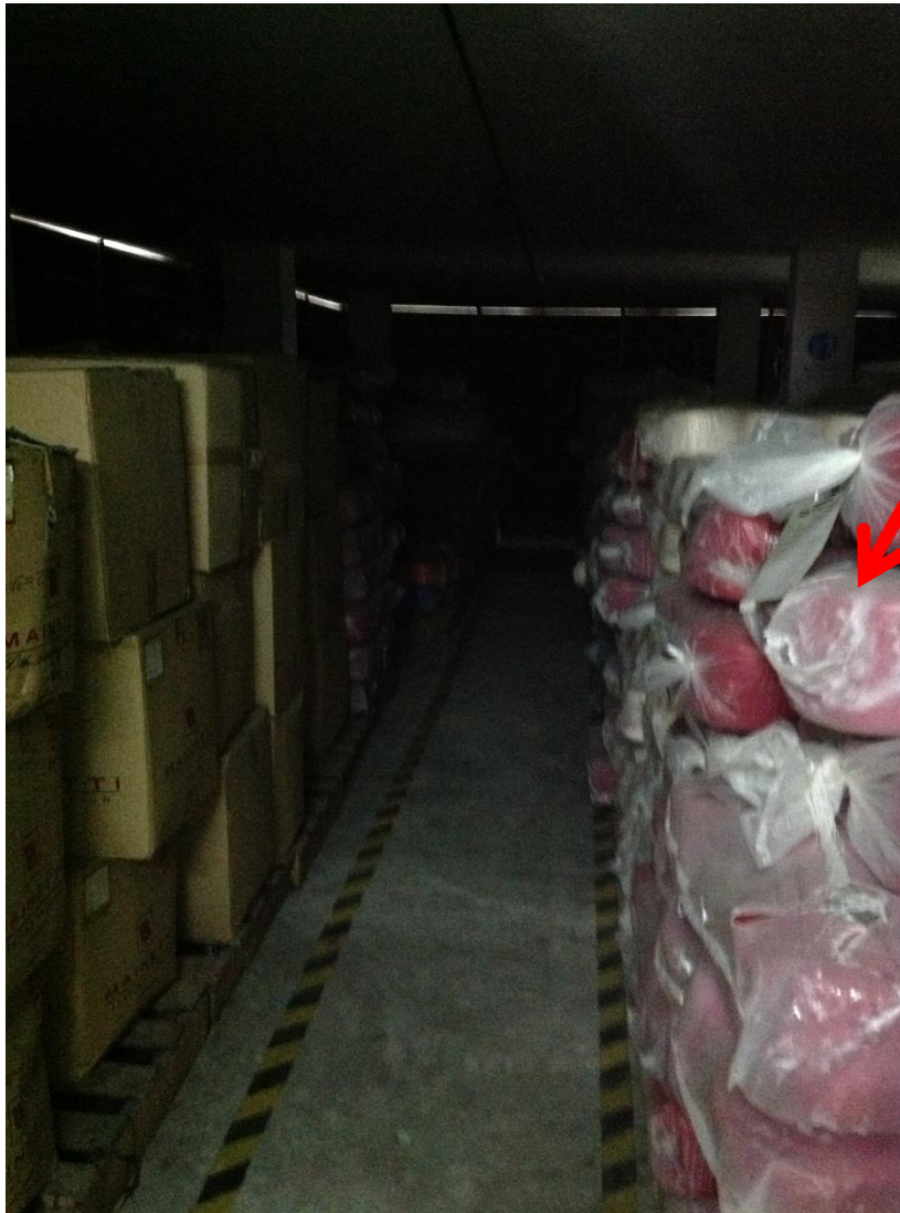
Excessive loading in Temporary Yarn Store on 5 th Floor
