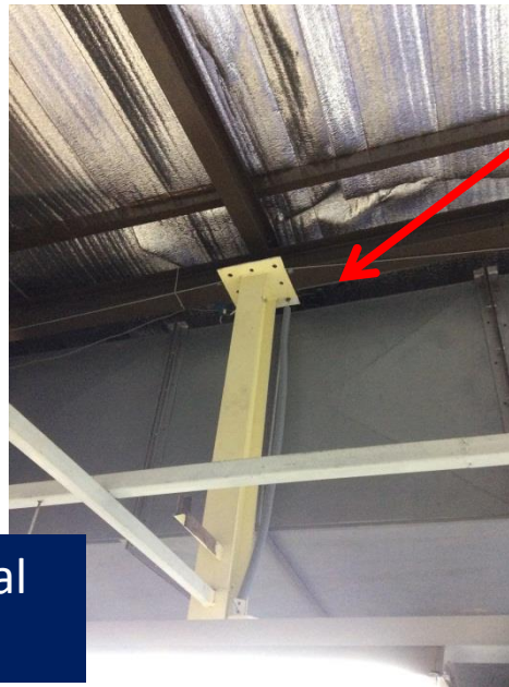
Engineer to review adequacy of structure to carry water tank
