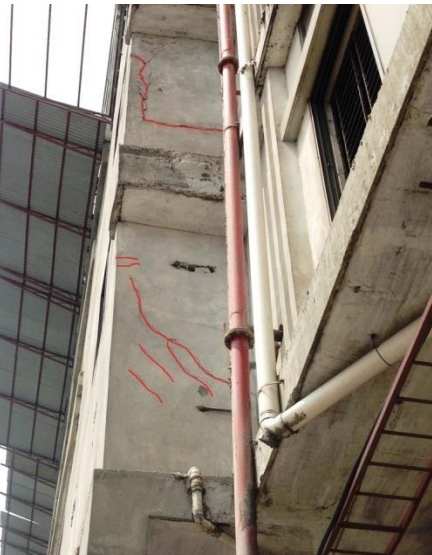
South Side Cantilever Area
