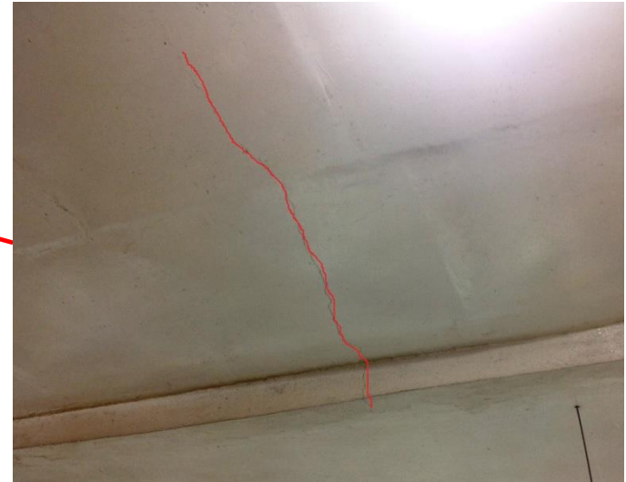
2 nd Floor At the front of stair case
