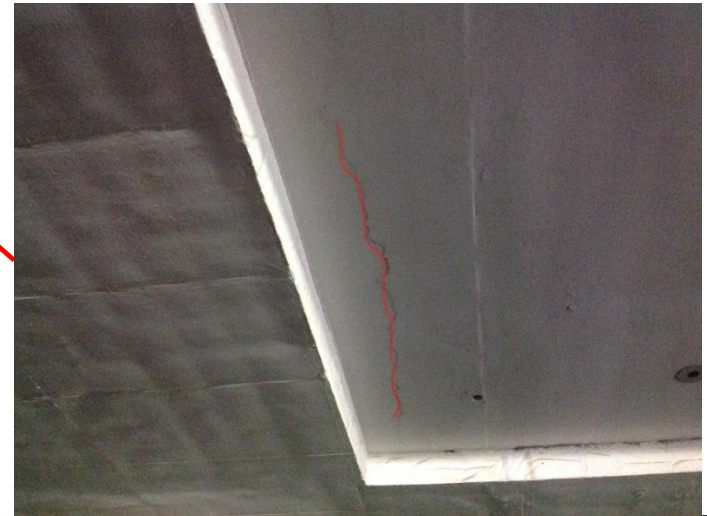
Basement below GF Washing Plant Area
