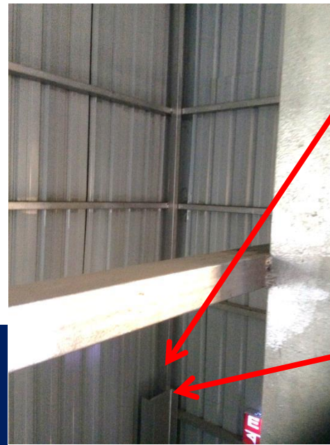
Façade of Chemical Store is tack welded to top of column.
