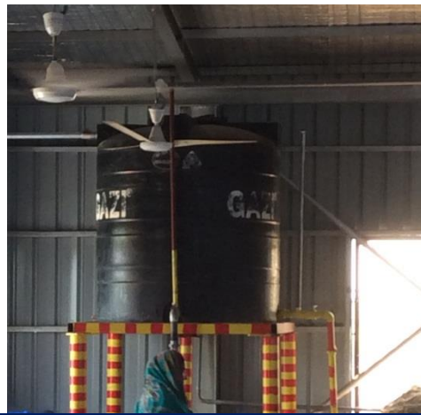
Engineer to review adequacy of structure to carry water tank
