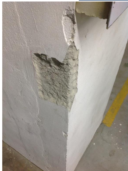
Tested Ground Floor Column – Stone Chips
