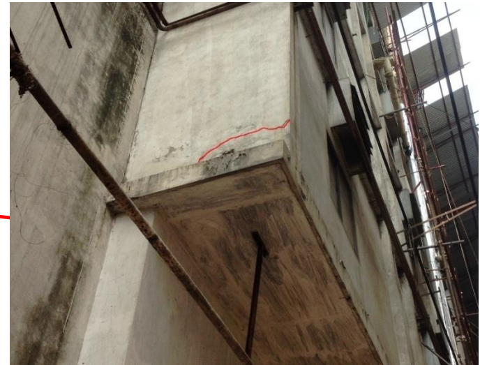
East Side Cantilever Area
