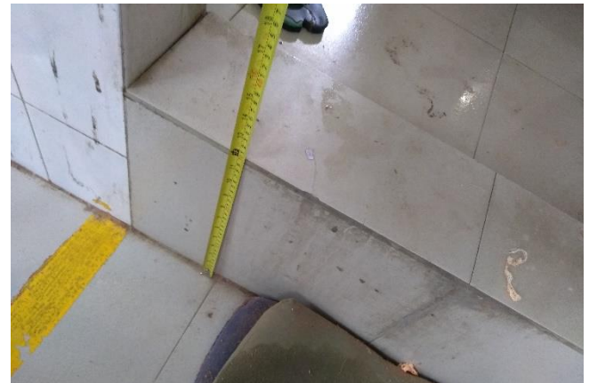
Toilet Build up
