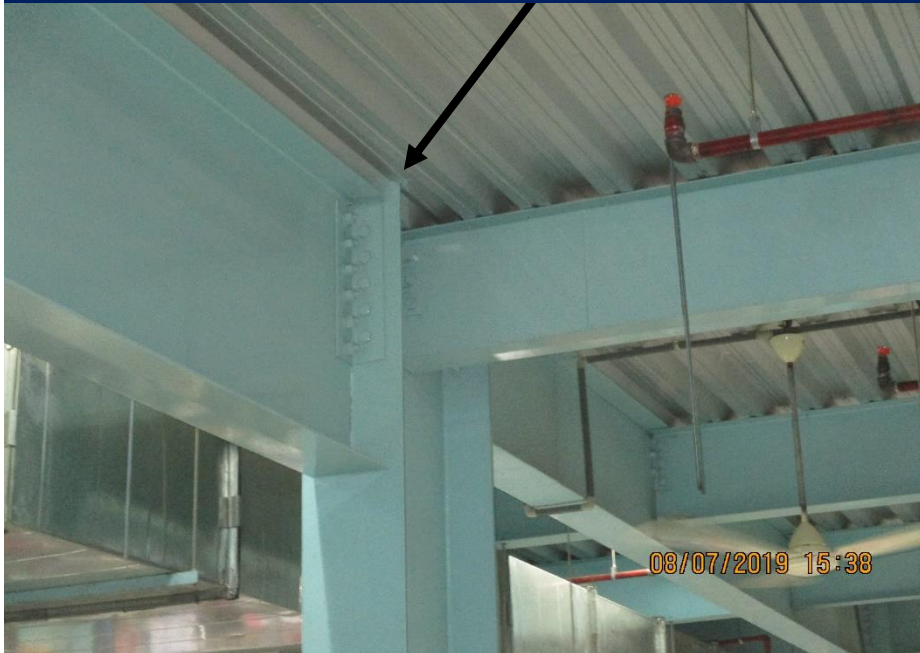
Partially fixed in N-S/ Short Direction
