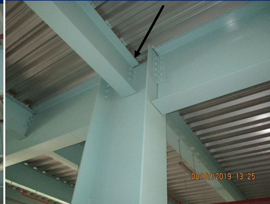
Pin/hinge Connection in E-W/ Long Direction
