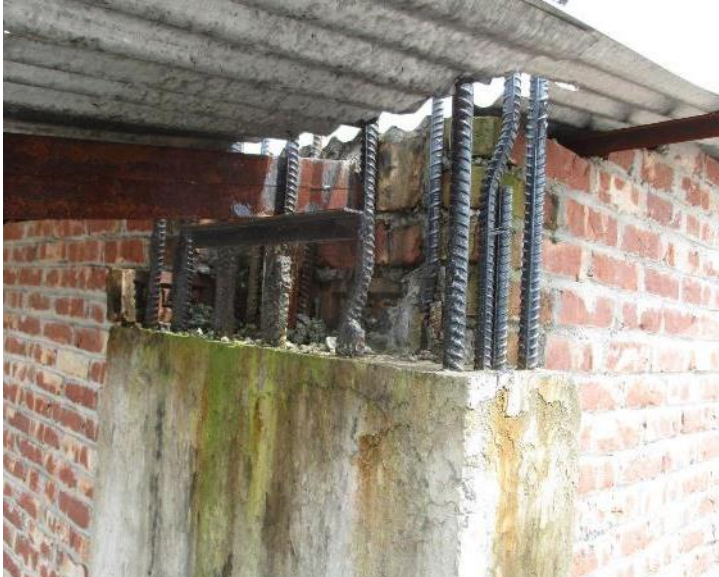
14 rebar observed in C1A column at grid G-4
