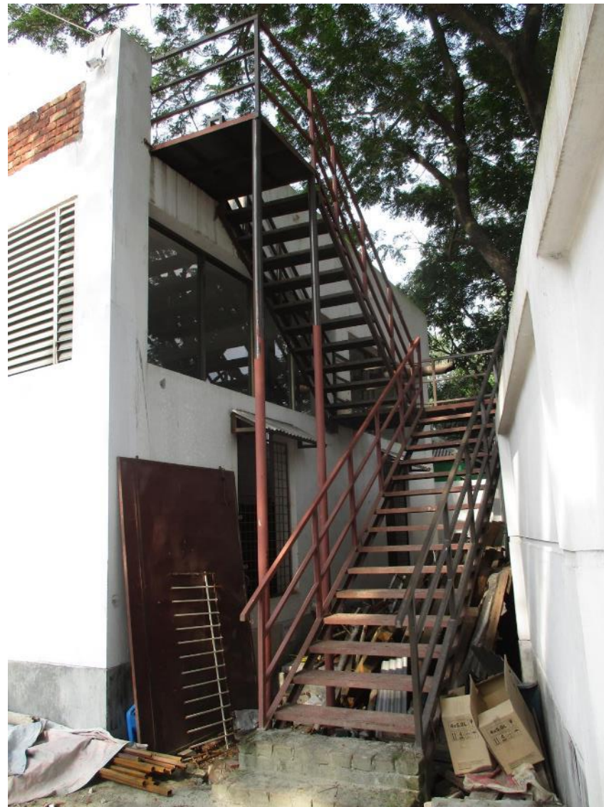
Steel stair adjacent to Utility Building
