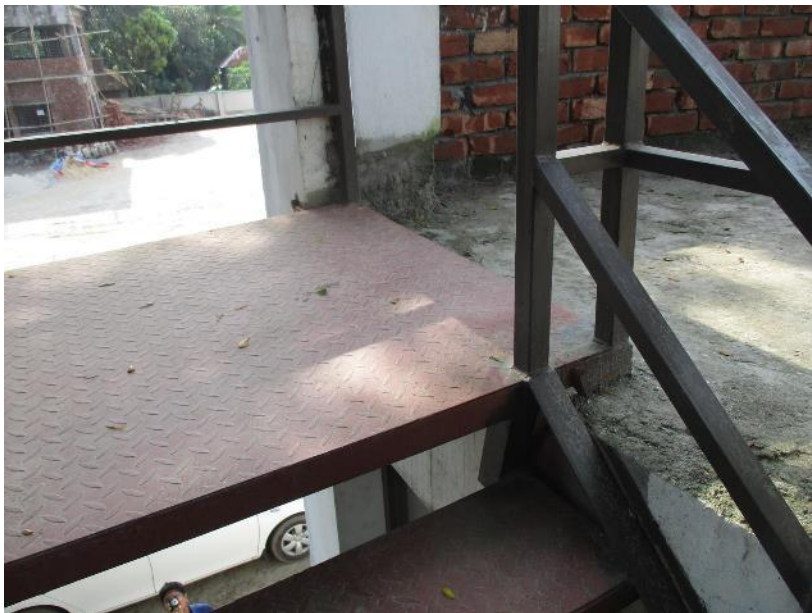
Connection between steel stair and Utility Building
