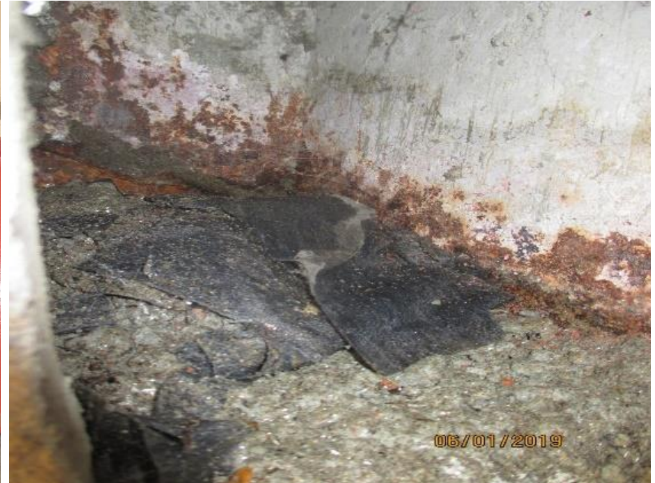
Corrosion in steel members at stair zone.
