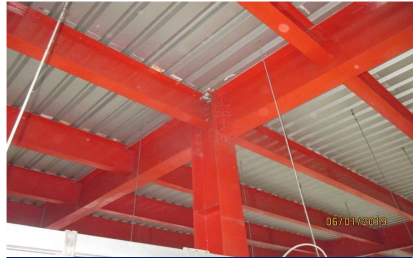
Sub-beam on site
