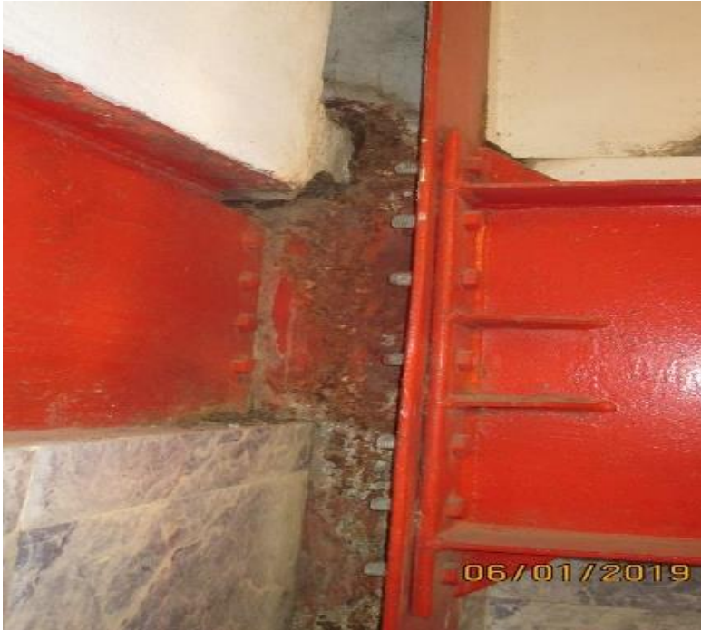
Corrosion in steel members at stair zone.
