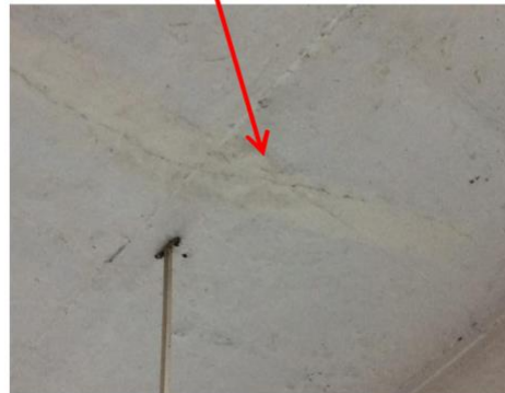
2 nd floor slab soffit
