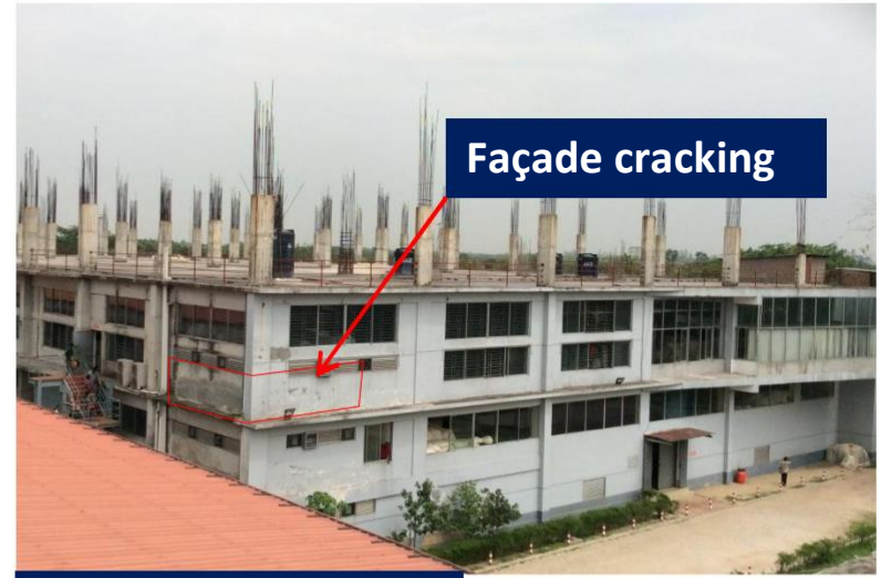
Façade cracking
