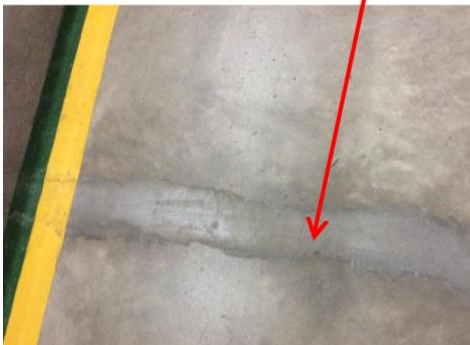
1 st floor slab
