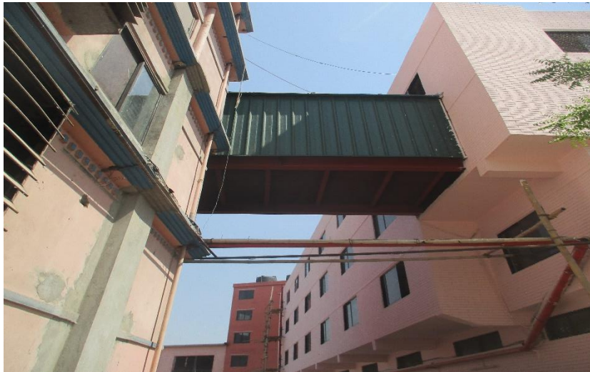
Connecting bridge was found on the north side of the building.
