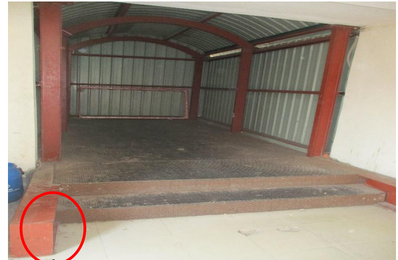
Steel beam and column of the connection bridge
