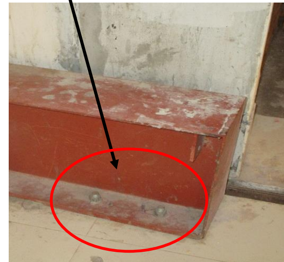
Steel beam was bolted with RC beam of the building
