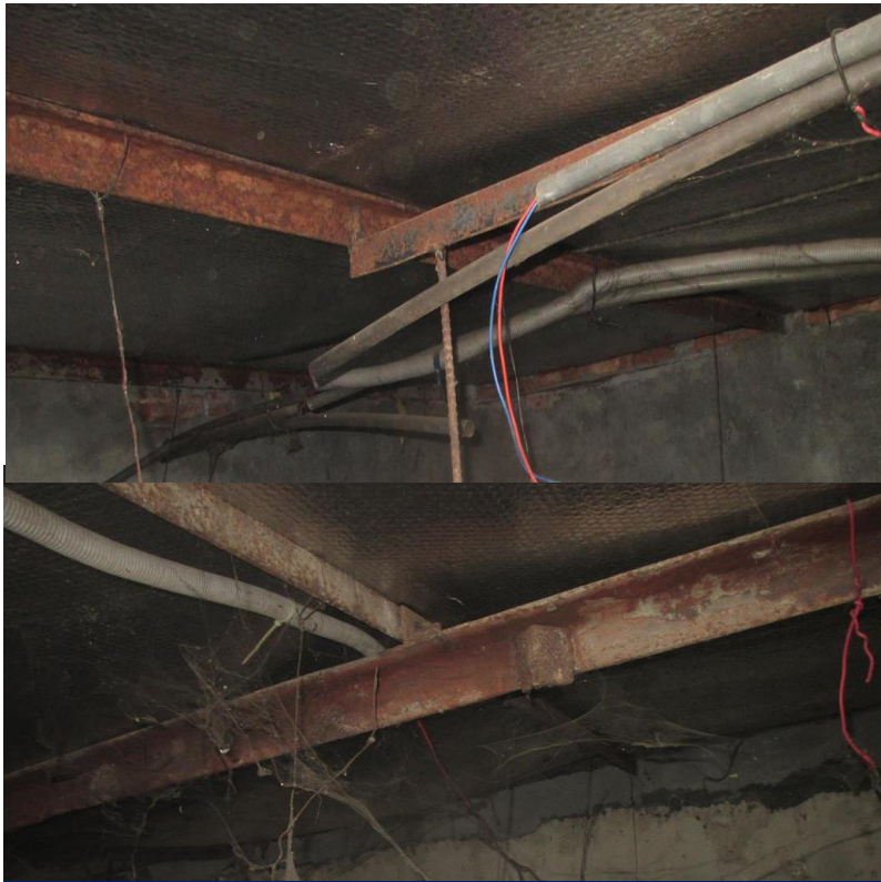
Non-engineered roof shed
