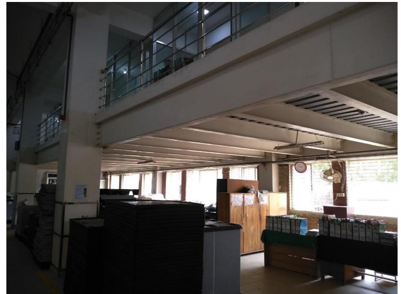
Mezzanine Steel frame connected with RC column of factory building
