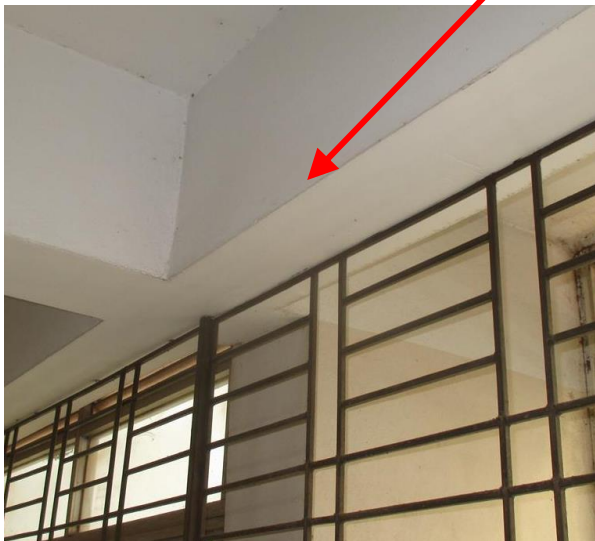
Eccentric connection at beam-column joint (marked Locations)
