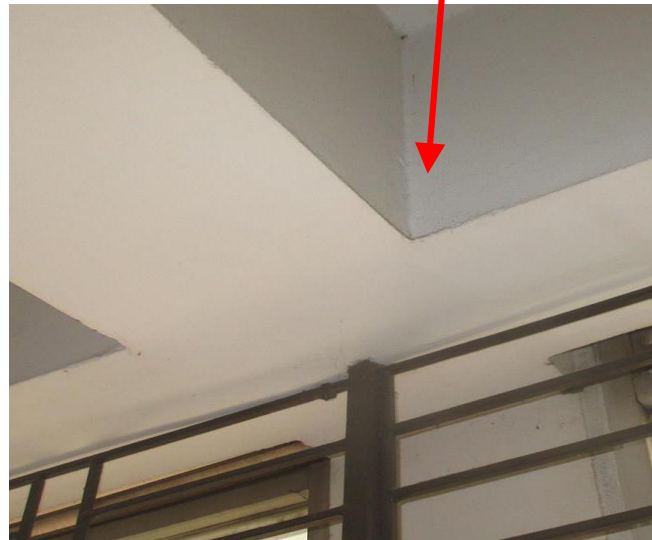
Eccentric connection at beam-column joint (marked Locations)
