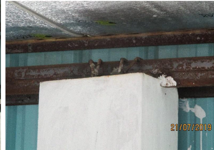
Non-engineered connection
