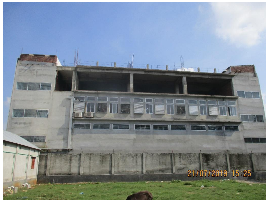
3-storied Main Building with a mezzanine
