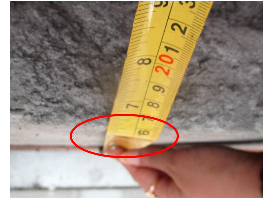
6 inches cantilever slab
