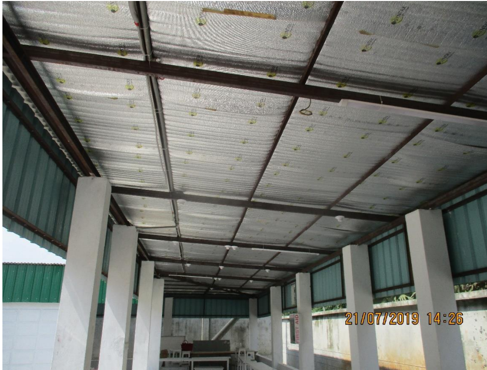
Light weight roof supported on RC column
