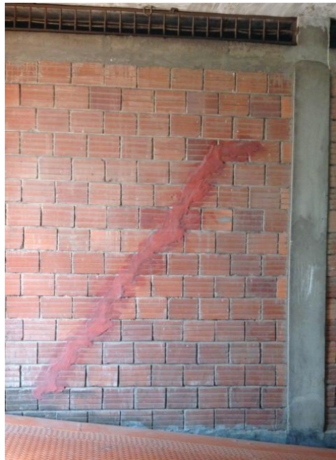
Crack in partition – 2nd floor
