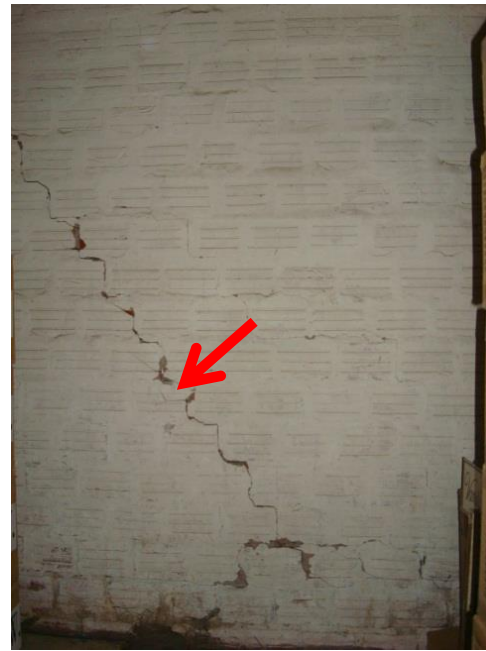
Crack in partition – 2nd floor
