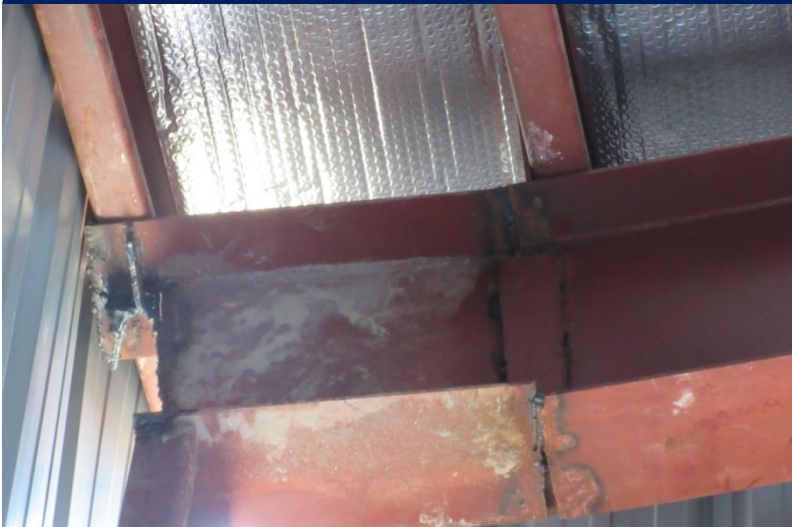
Non-engineered joint.
