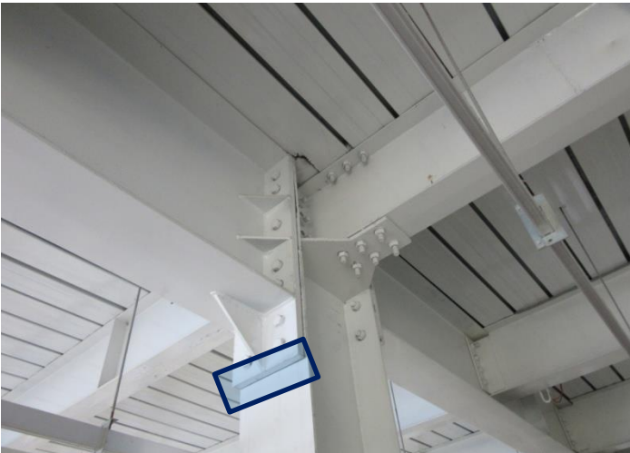
Some of the connections between different steel members were non-welded
