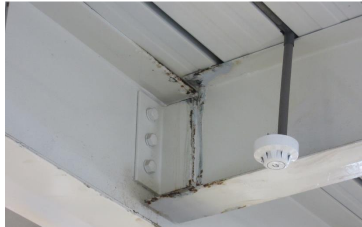
Rusting observed in some of the steel elements as well as not a full contact on the connections plates.
