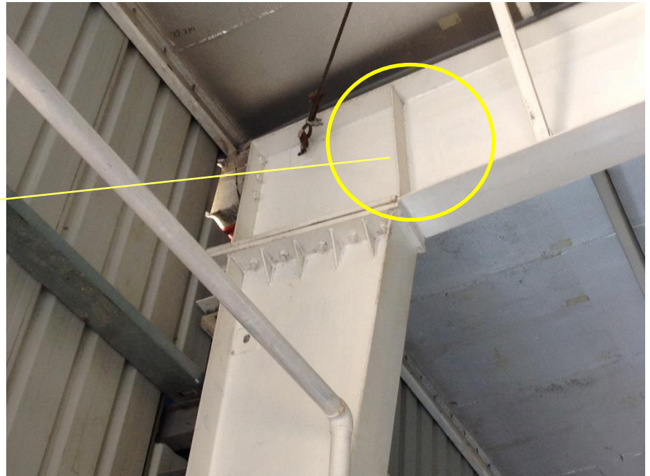
Steel member with rib to transfer vertical load to supporting column
