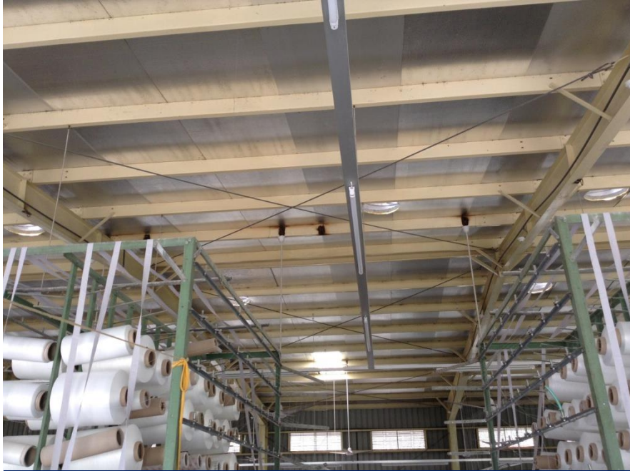
Most of the bracing are apparently not sufficiently tight
