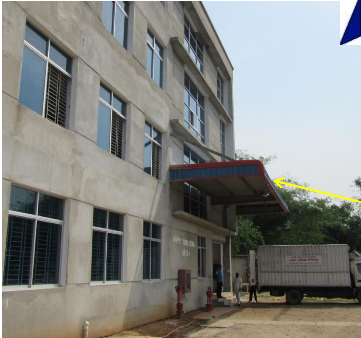
Apparently non-engineered canopy
