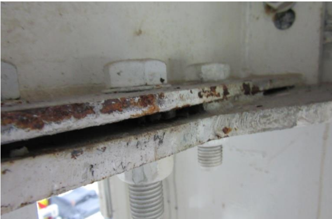
Rusting observed in some of the steel elements as well as not a full contact on the connections plates.
