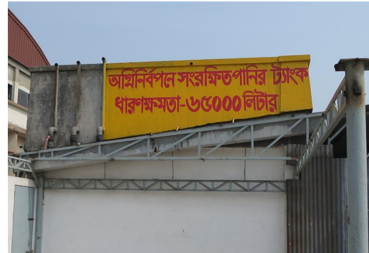
65,000 Litre R.C Water tank (1)
