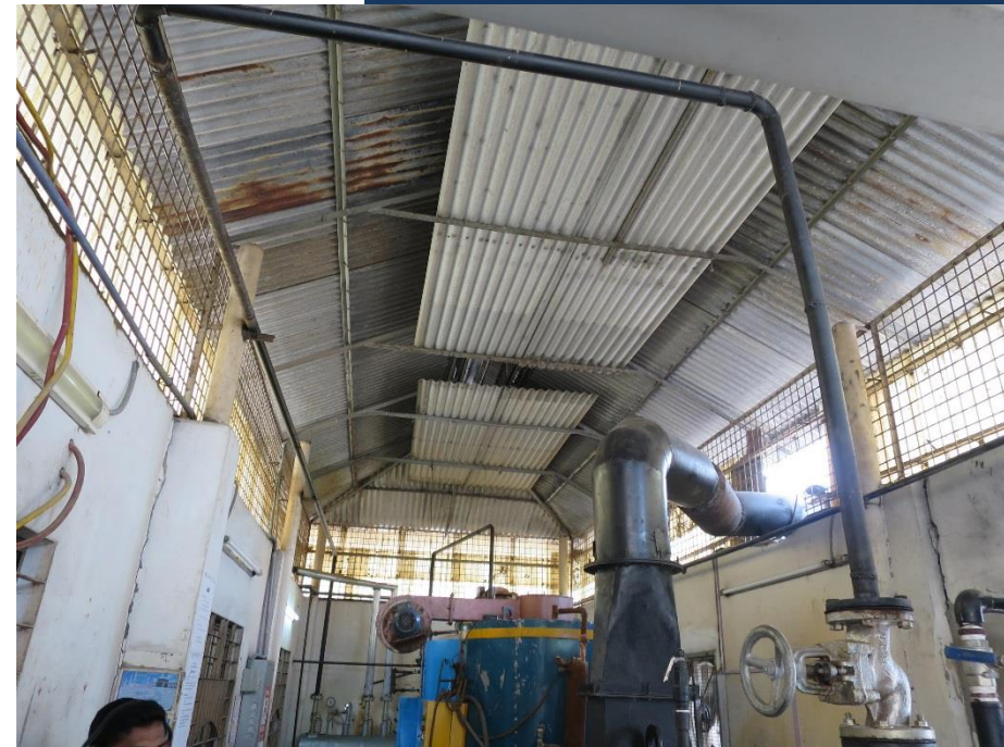
Boiler House Shed
