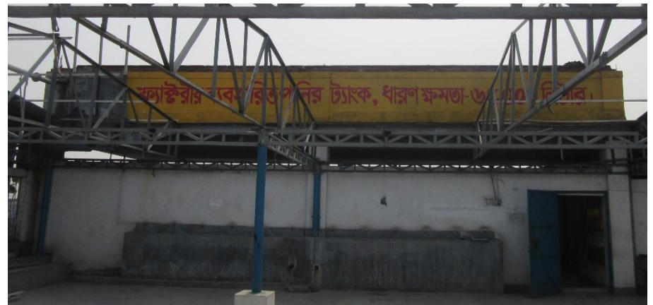
65,000 Litre R.C Water tank (2)
