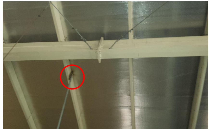
Lack of roof bracing struts and non-engineered hangers (welded to purlins )
