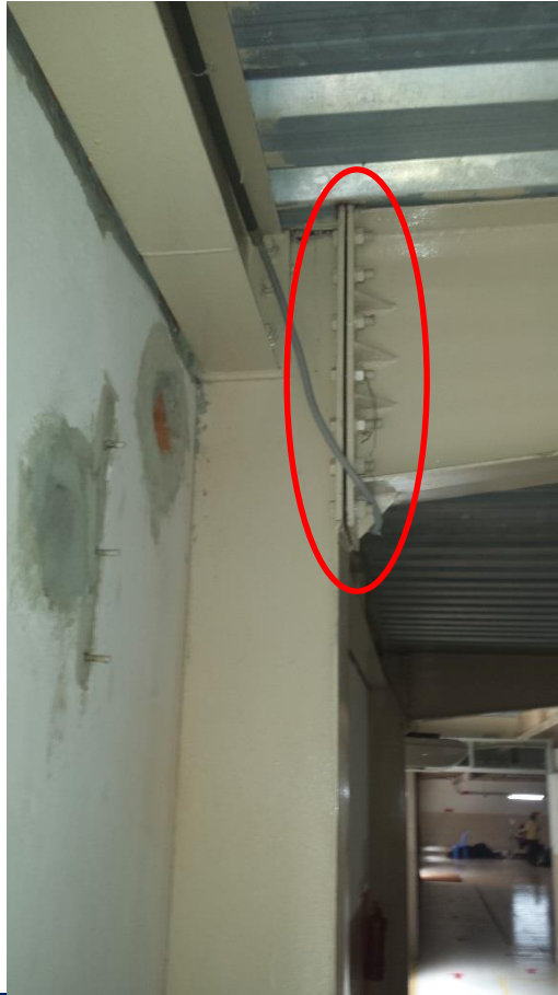
Building 1 – 1 st Floor main beam/column connections – gaps between endplates
