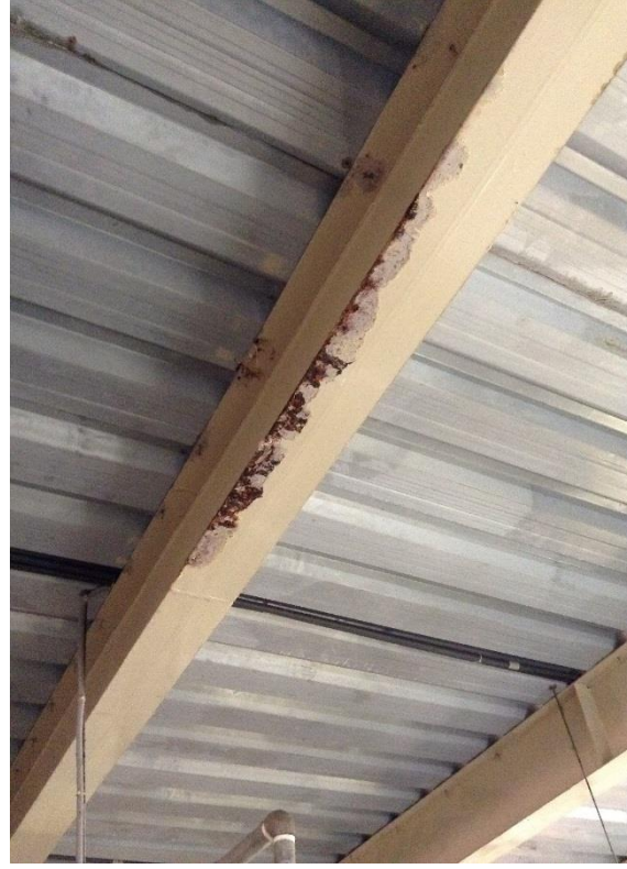
Building 1 - corrosion in 1 st floor beams
