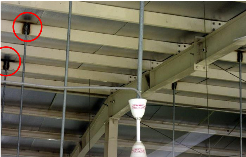
Lack of roof bracing struts and non-engineered hangers (welded to purlins )
