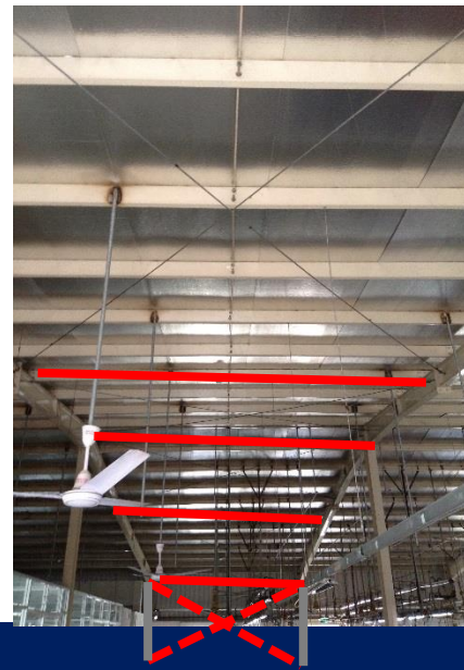
Lack of roof bracing struts and vertical bracing
