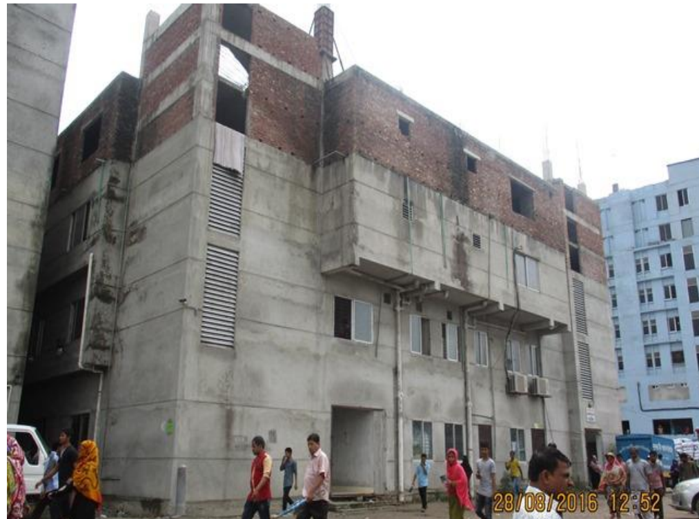
Factory Building 4 storied
